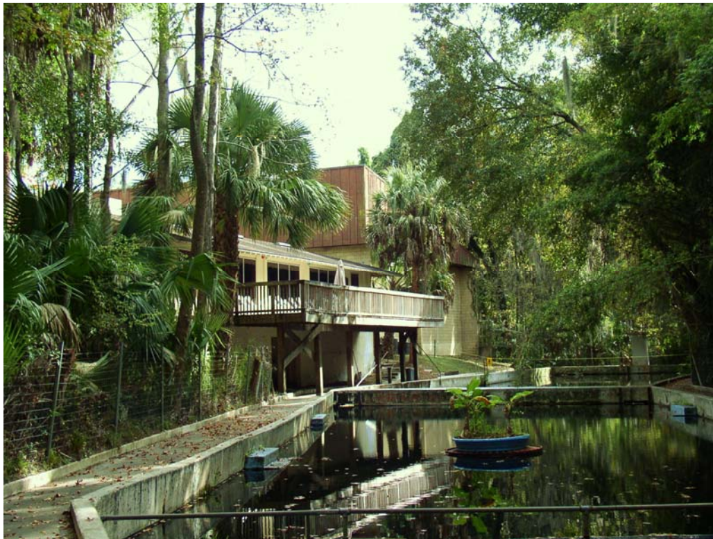
FIGURE 5. VIEW OF GLEN SPRINGS CLUBHOUSE AND CURRENT ELKS LODGE. (PHOTO BY A. GROSSMAN, 11/22/2012)
