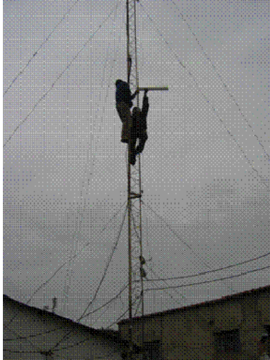
Figure Anx.3.4: Installation of Yagi (directional) antenna
