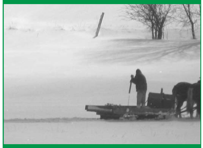
A regular T-bar post pounder made out of an old hydraulic cylinder and an 8-inch (200-mm) solid steel plug was used to pound the posts into the frozen soil under the snow.
