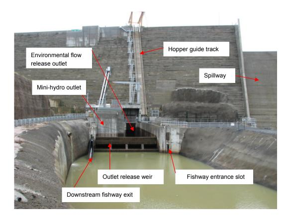
Figure 3 Upstream fishway entrance and layout of dam infrastructure (looking upstream)
