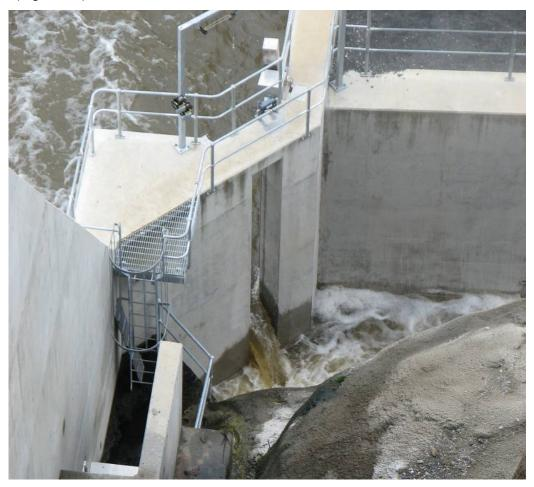
**Figure 21** Fishway entrance slot (spillway) with reverse flow during a 170mm spillway flow and environmental outlet release of 40 cumecs 3<sup>rd</sup> March 2010.
