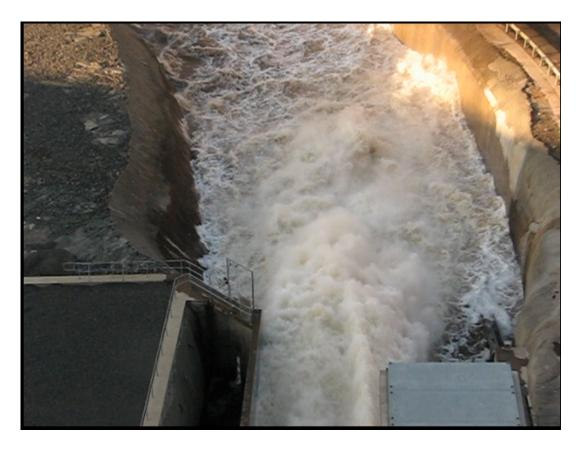
**Figure 18** Flow conditions downstream of the fishway entrance slot during an environmental outlet release of 40 cumecs.
