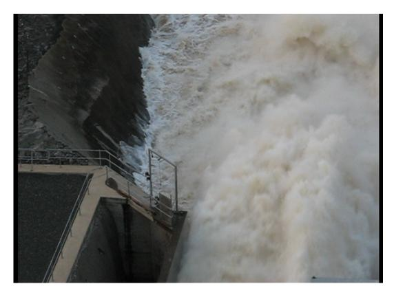
**Figure 19** Flow conditions downstream of the fishway entrance slot during an environmental outlet release of 60 cumecs.
