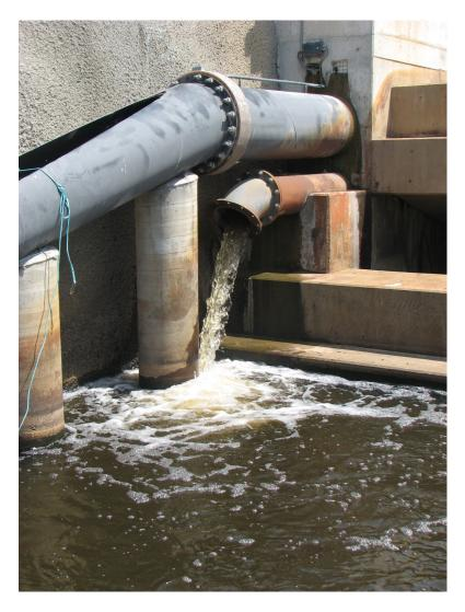
Figure 24 Downstream fishway outflows during attraction phase in the outlet release channel.
