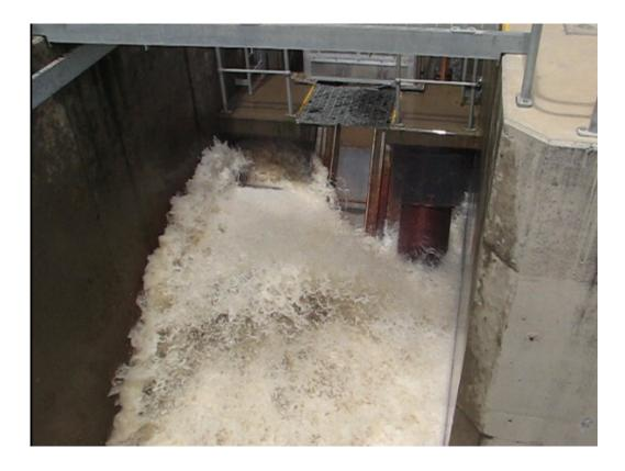
**Figure 22** Flow conditions at fishlift entrance slot during increased supplementary attraction flow (Left supplementary diffuser valve at 100%, Right supplementary valve at 7%).
