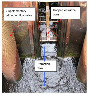
Figure 6 The hopper set in attraction phase within the hopper chamber.
