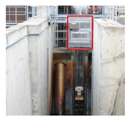
Figure 23 Quad leaf gate arrangement at the fishlift entrance slot, red outline shows the screen over the gate hoist.
