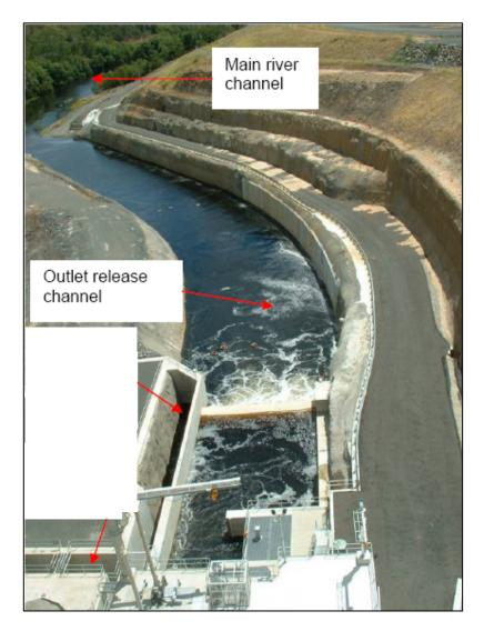
Figure 1 Paradise Dam outlet release channel and fishway approaches (looking downstream).
