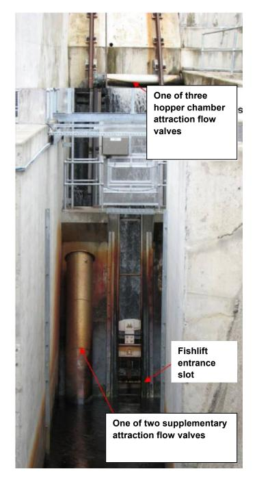
**Figure 2** Entrance to the fishlift and attraction flow valve arrangement (looking upstream from within the fishlift approach channel)
