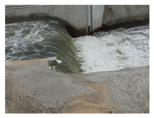
**Figure 17** Flow conditions downstream of the fishway entrance slot during an environmental outlet release of 20 cumecs.
