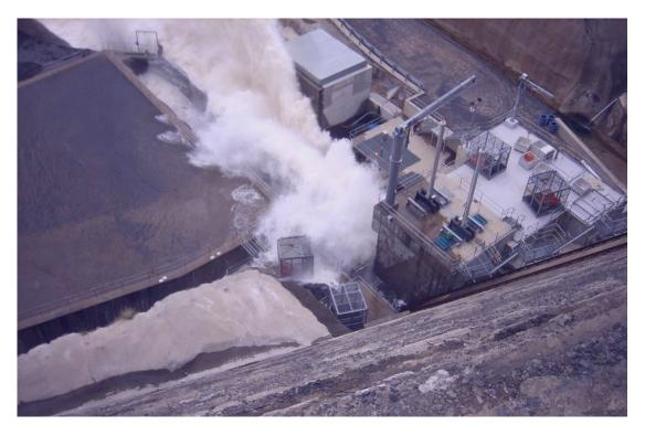
**Figure 20** Flow conditions in the fishway entrance slot during an environmental outlet release of 240 cumecs and 120mm spillway flow 23<sup>rd</sup> September 2010.
