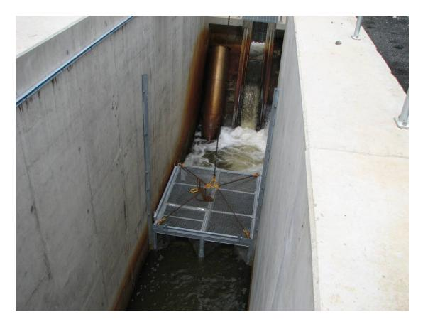
Figure 5 The upstream trap set in place within the fishlift approach channel.
