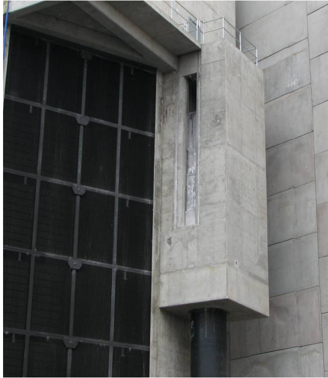
Figure 2 The downstream fishway prior to filling of the dam showing the fishway entrance slot, the fishlock chamber and the standpipe. Note the adjustable quad leaf gate in the fishway entrance slot.
