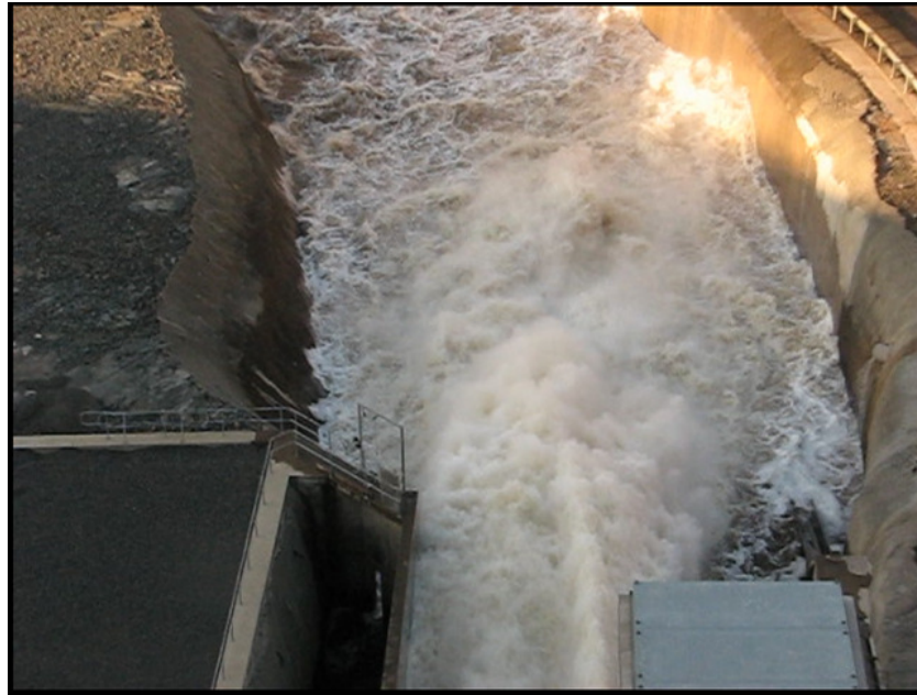
Figure 34 Fishlock exit conditions during an environmental outlet tower release of 40 cumecs. N.B. Fishlock exit chute is shown in the bottom right corner of the image.
