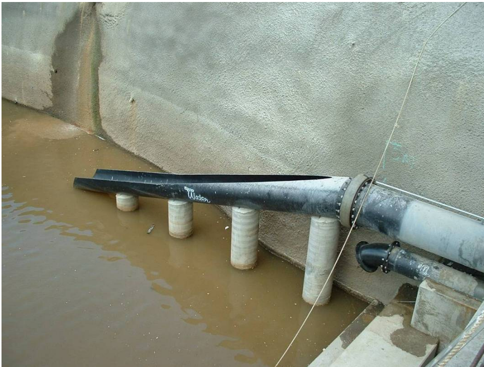
Figure 2 The downstream fishway prior to filling of the dam showing the fishway entrance slot, the fishlock chamber and the standpipe. Note the adjustable quad leaf gate in the fishway entrance slot.
