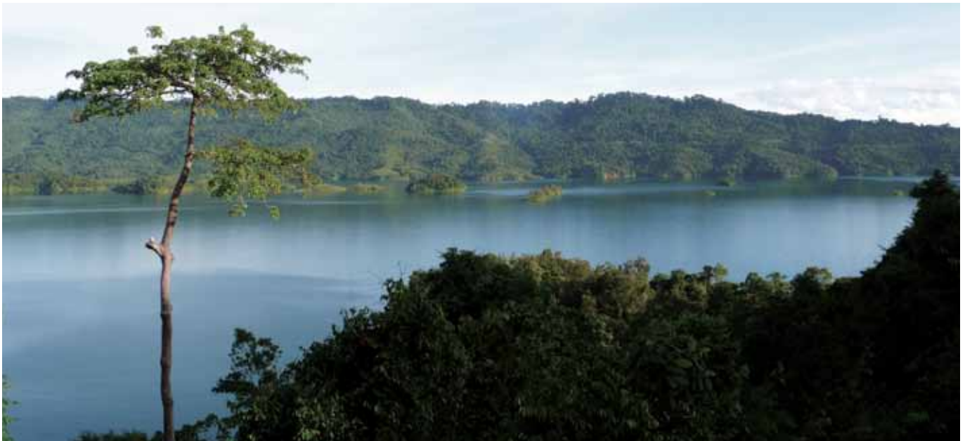
Figure 11: The view from the Hilton Batang Ai Longhouse sitting on the reservoir of the Batang Ai Hydroelectric Dam
