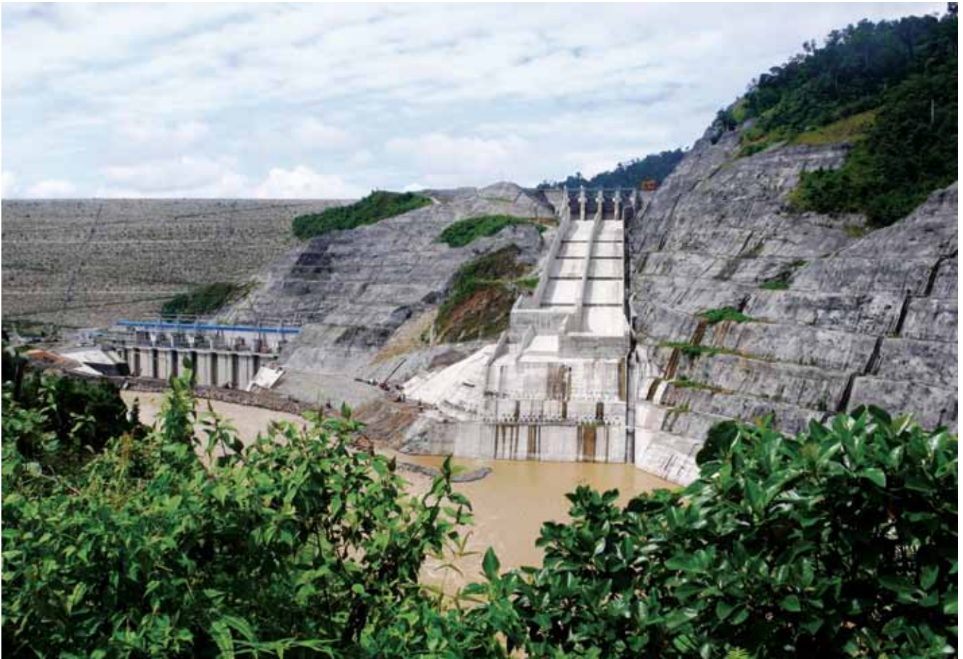
Figure 5: The 2,400 MW Bakun Dam (near completion), July 2010
