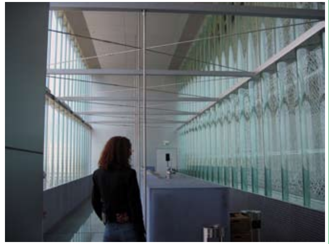
Fig. 3. In between the two corrugated glass walls a bar, a glass one of course, was made. In the air the trusses that take up the wind load on the façade.
