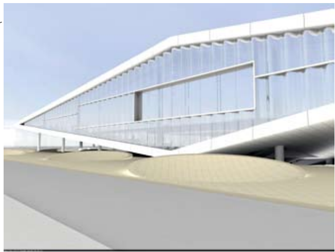
Fig. 10. External view of the Qatar corrugated glass facade
