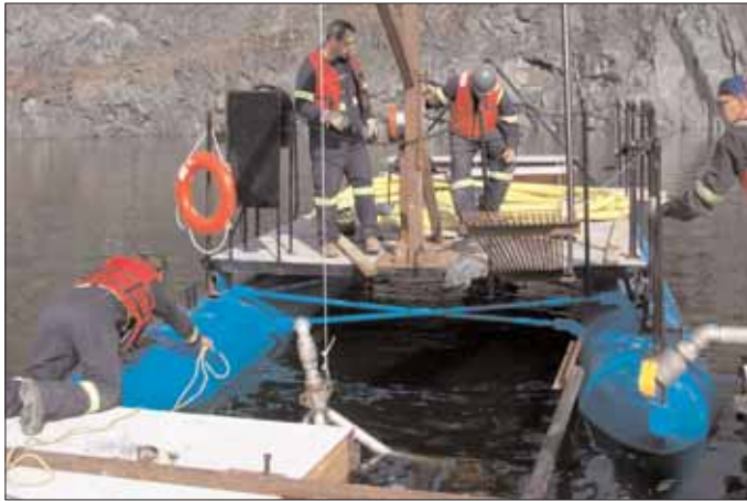
Installing the diffuser in the Zone 2 Pit.
