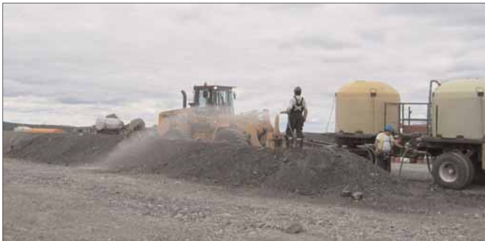
Watering a windrow in the waste oil lay-down area to increase moisture content.
