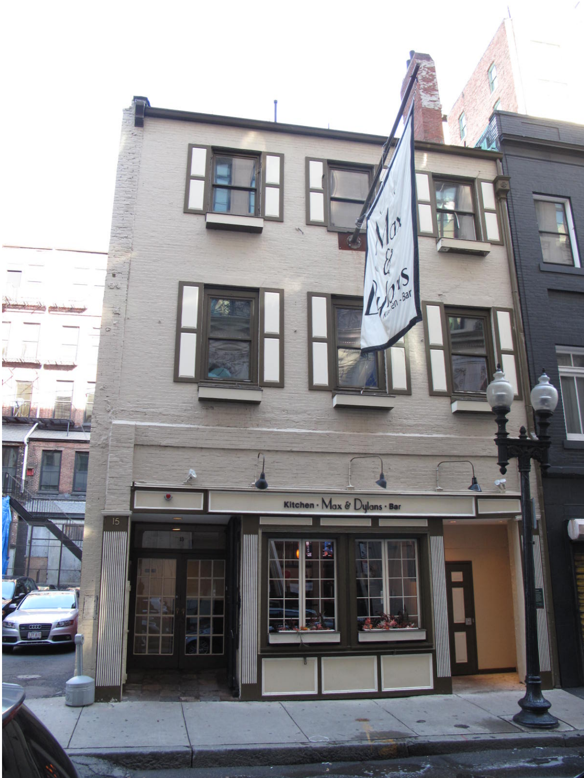
Figure 1. 13-15 West Street, 2010. (Larson Fisher Associates)
