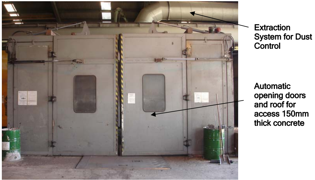
Figure 20: Existing noise enclosure that surrounds the shakeout machine
