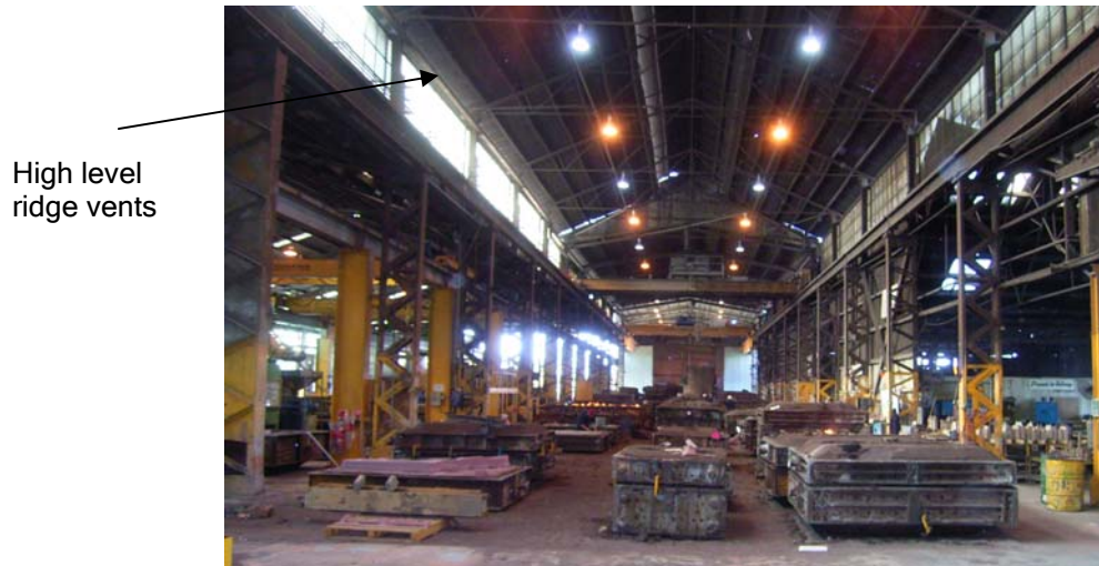
Figure 12: Current foundry building. Note the ridge vents at the roof line associated with the natural ventilation system..
