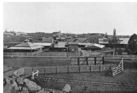
Mabel Mill of the New Ravenswood Co. c1902.
