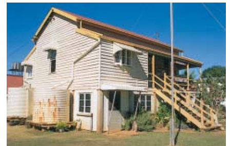
96. Former telegraph office at Mount Surprise.
