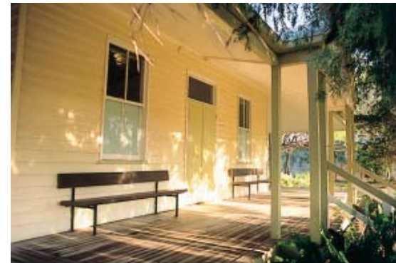
35. Court house verandah.
