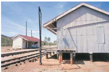
126. Chillagoe railway station and goods shed.
