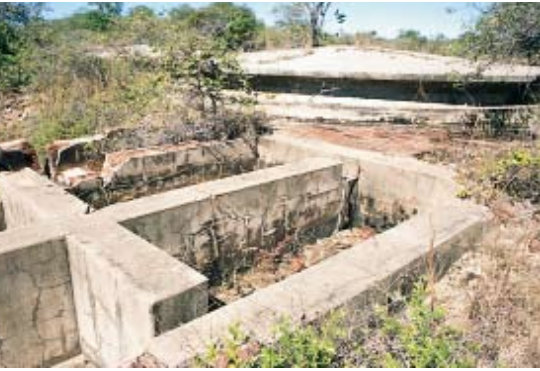
19. Great Extended Mill foundations, Totley.
