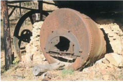
153. Cornish boiler and stone bed at the Comet.
