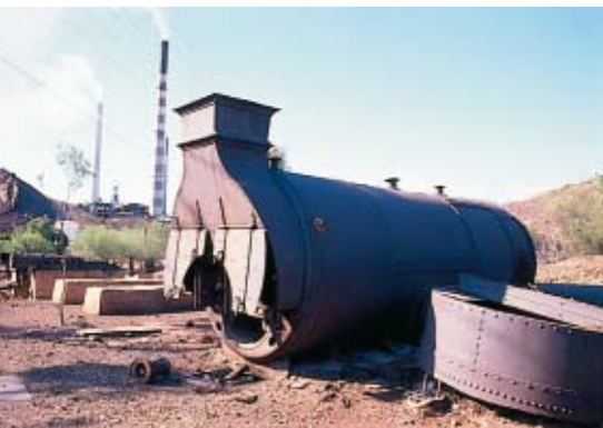
48. Lawlor Shaft boiler and haulage foundations.
