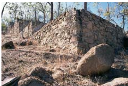
141. Foundations of the Corporation's mill.
