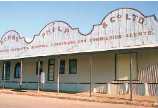
57. Former Burns Philp and Co. store.
