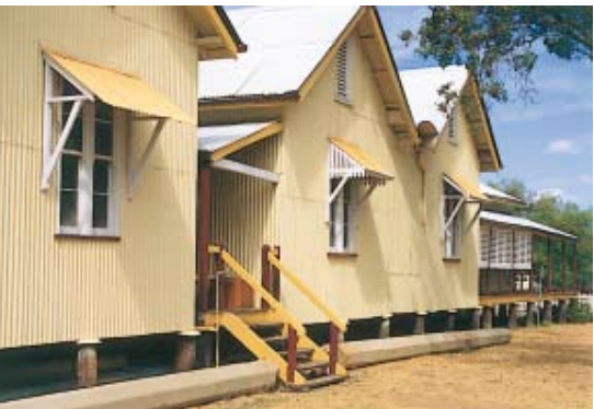
73. Former court house.
