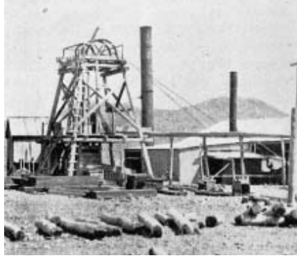
137. Tyrconnel Mine headframe, c1922.
