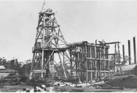
48. Lawlor headframe under construction, 1929. (Courtesy of John Oxley Library)
