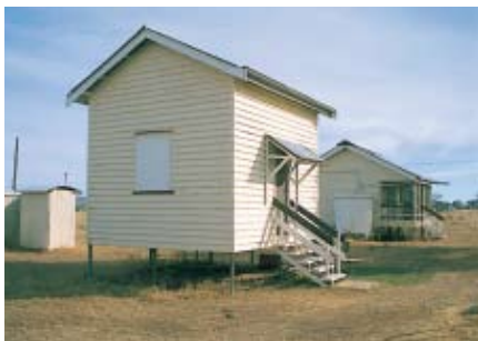
91. Tracker's quarters and police station.
