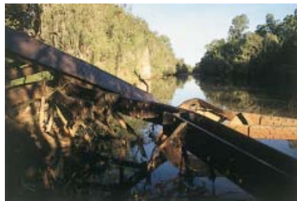
156. Railway bridge ruins, Laura River.
