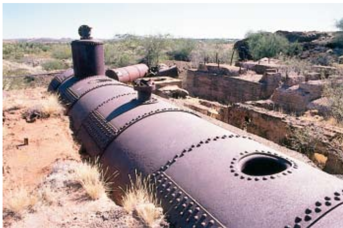
32. Cornish boilers and haulage plant foundations.
