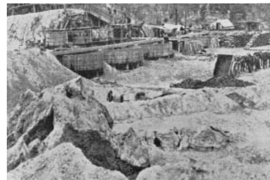
75. Treating the Cumberland battery dumps, c1904.
