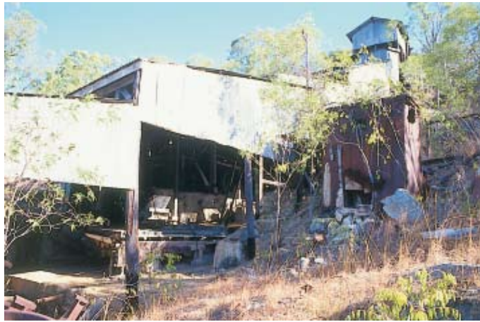
137. Tyrconnel battery shed.
