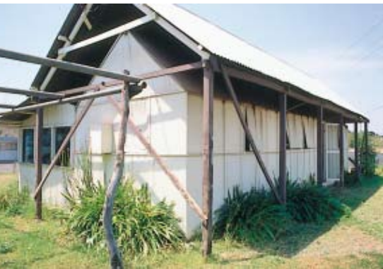
51. Former miner's tent house at Mount Isa.
