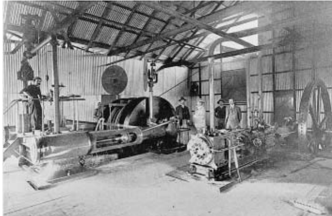
14. Ravenswood Deep Mine winding plant, c1905.
