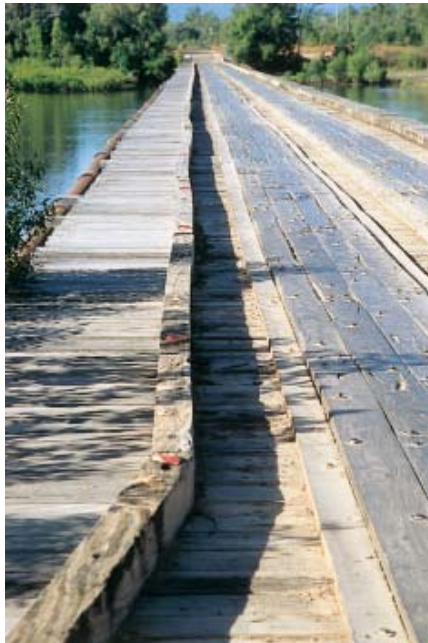
163. Annan River bridge.
