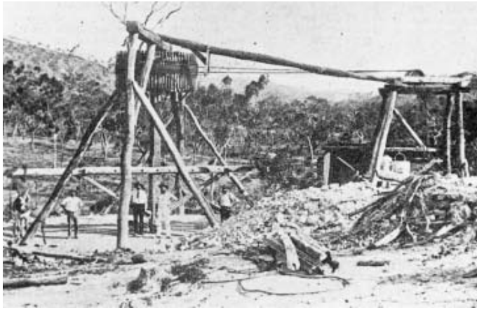
159. Horse whim at the Great Northern Mine c1896. (Courtesy of John Oxley Library)
