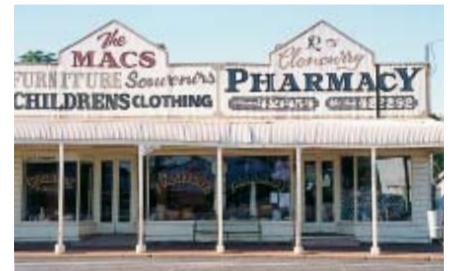
34. Former A.J. Smith and Co. store.
