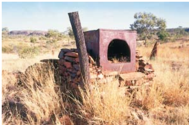
53. Hotel bake-oven, adapted from a water tank.
