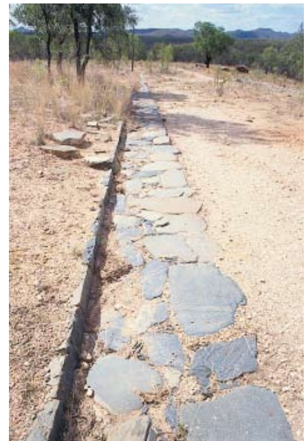
152. Stone kerbing on Leslie Street, Maytown.
