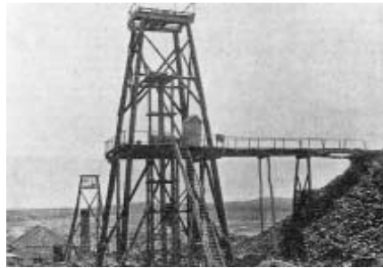
12. General Grant Mine headframe, c1901.
