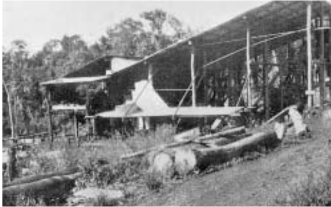
162. Gordon's Battery at Iron Range, c1937.
