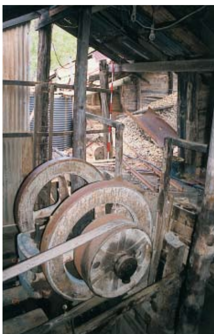
121. Jaw crusher and ore bins, Emuford Battery.
