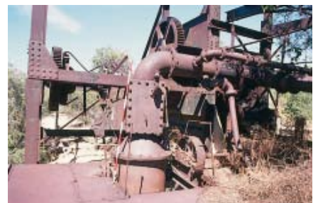
158. Gold dredge pump and bucket drive.
