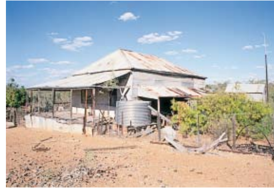
94. Battery manager's house at Kidston.
