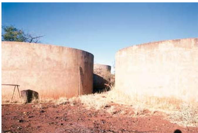
33. Leaching vats at the Metallurgical Plant site.
