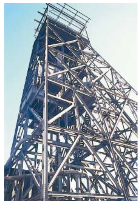
47. Steelwork of the Urquhart Shaft headframe.
