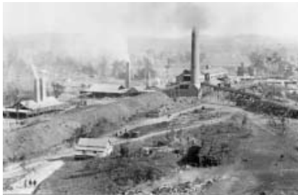
99. Mount Garnet copper smelter, c1902. (Courtesy of John Oxley Library)
