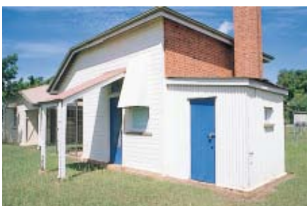
142. Former assay office at Mareeba.
