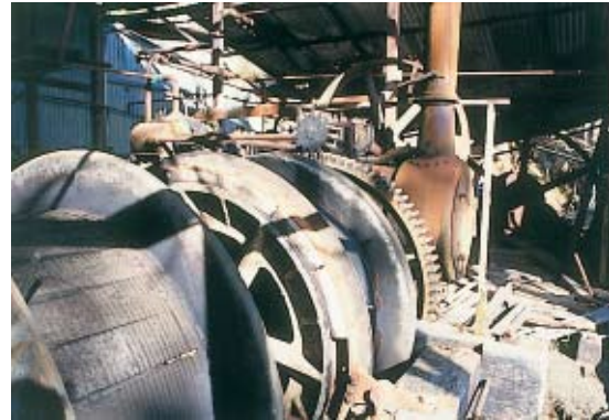
103. Haulage plant at the Eastern Shaft.
