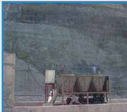
Slope stabilization at Powerhouse back slope
