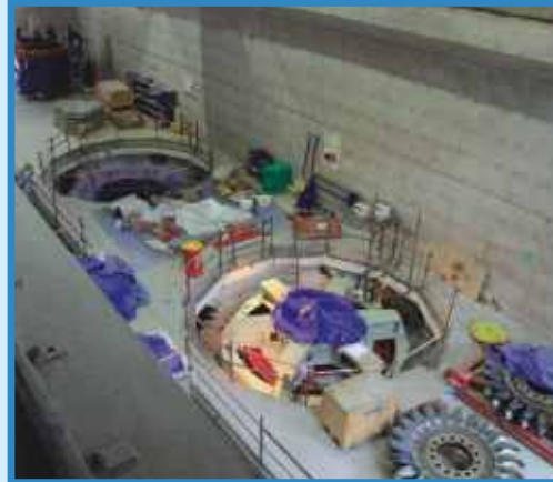
Erection bay of Power House
