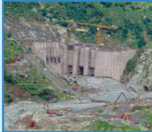
Visage of under construction Weir from upstream
