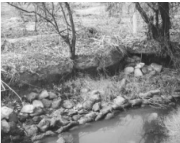
Rocks can be used to stabilise the toes of banks to limit erosion
