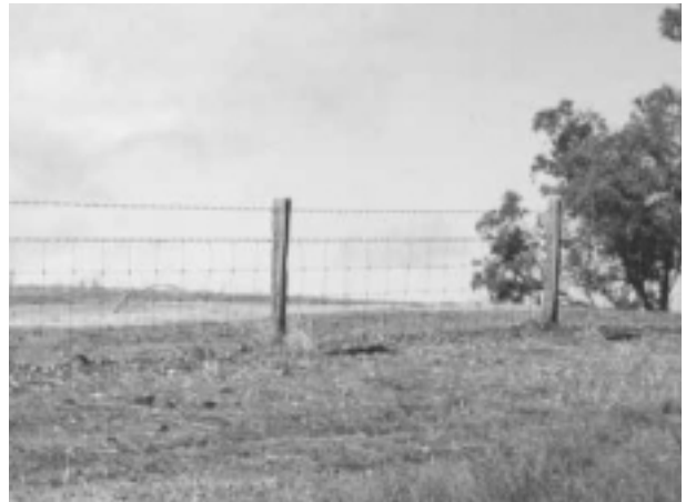
Fence condition: GOOD
