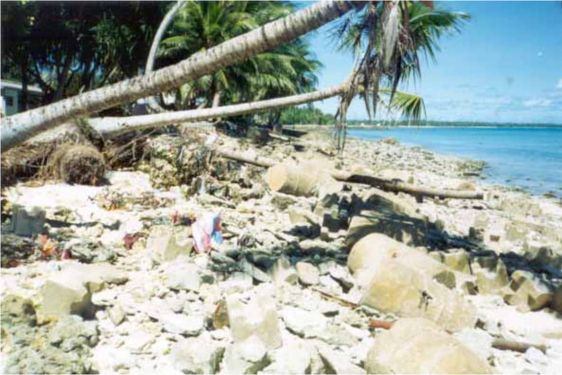
Figure 20. Coastal erosion to northeast of BS3. The shoreline of the reclaimed land in World War II is shown by the cemented coral stone cylinders, which were put in gasoline drums. The remains of a gabion basket seawall lie between the eroded coast and the cylinders.
