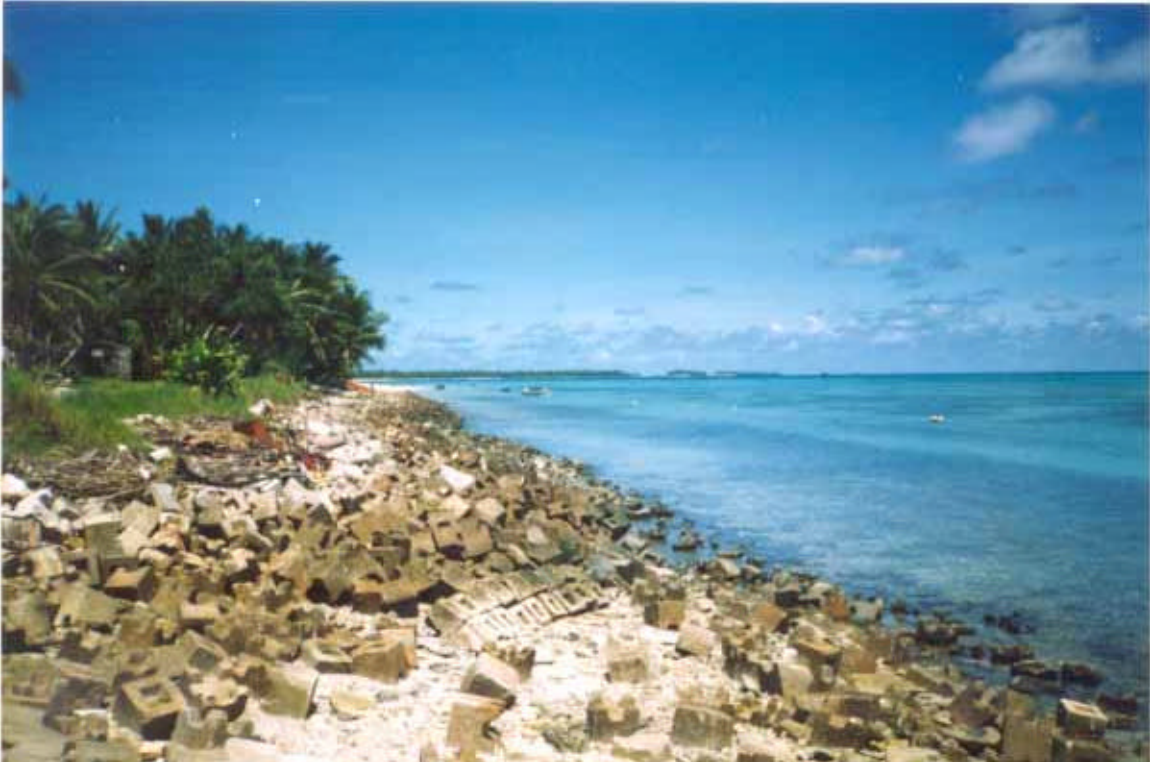
Figure 32. Piled concrete cubes forming seawall in the southwest of Catalina Ramp.
