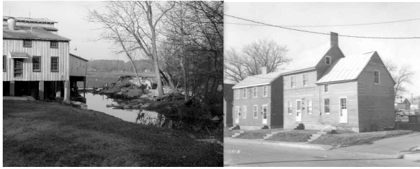
Fig. 21. Hearn and Rawlins Mill, after the dam washed out, S-213
