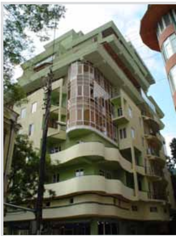
3. New construction in the Vera district (photo E. Kiladze)
