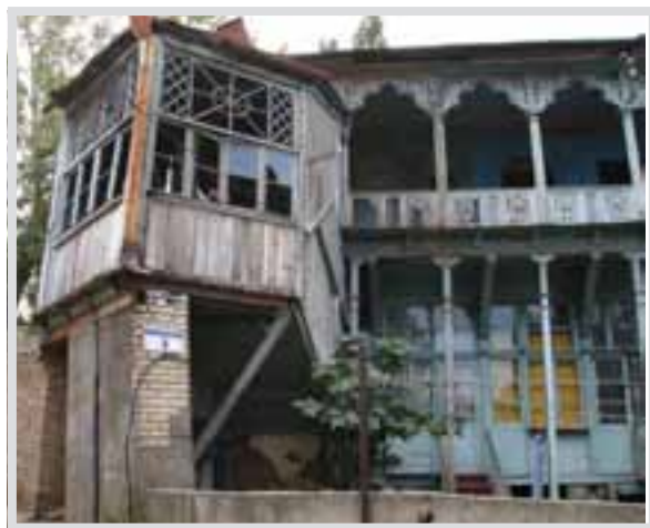
1. 3, Betlemi Street before restoration
