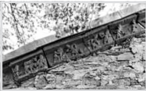
1. Korogo. Left part of the cornice.
