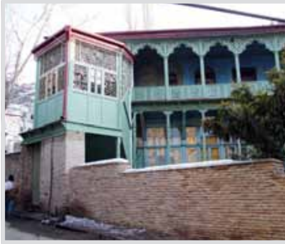
2. 3, Betlemi Street after restoration
