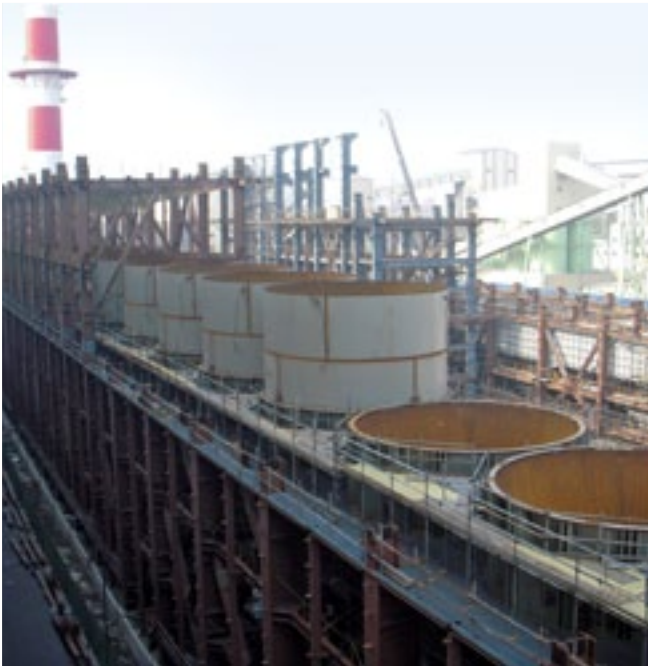
Proportioning bins under construction
