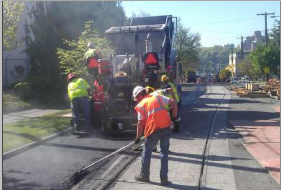
Asphalt paving on 14th between Yesler and Washington
