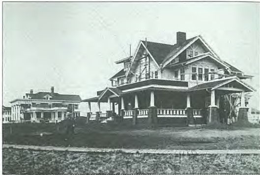
Ada Boulevard houses under construction, 1913. (GAI NA-1328-1136)
