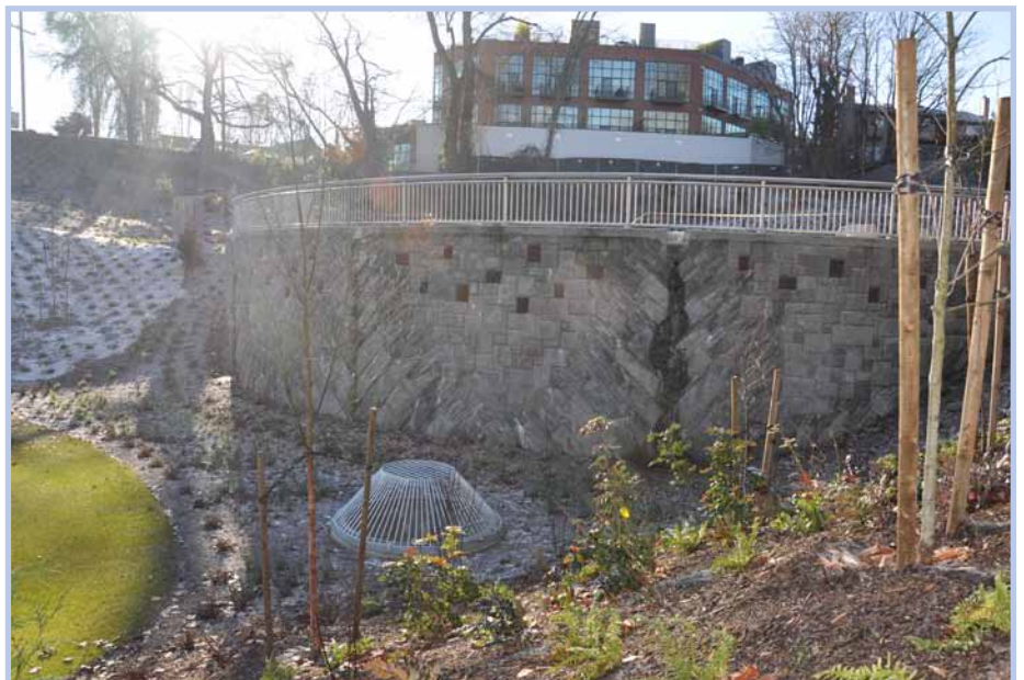
Phase 2 stormwater storage tank in Washington Park
