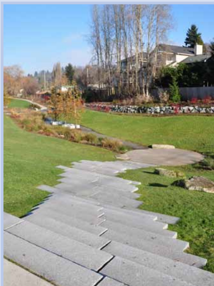
Stormwater holding area at 30th Avenue East and East John Street
