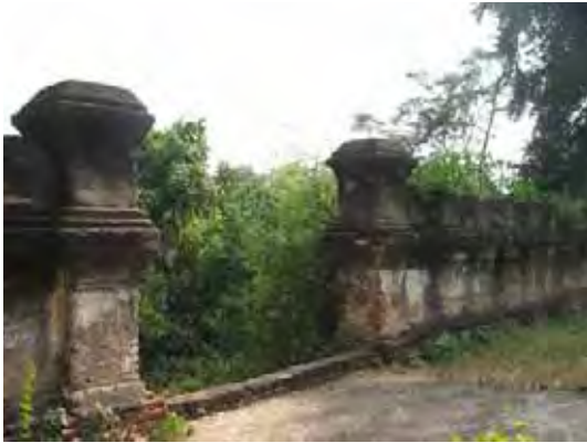
Figure 105: The boundary wall.
