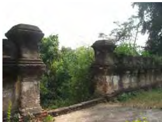
Figure 222: Condition of the wall.
