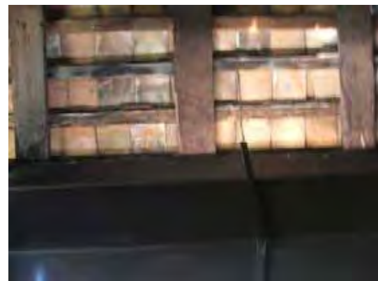
Figure 131: Terracotta tiles with a perlin hook.
