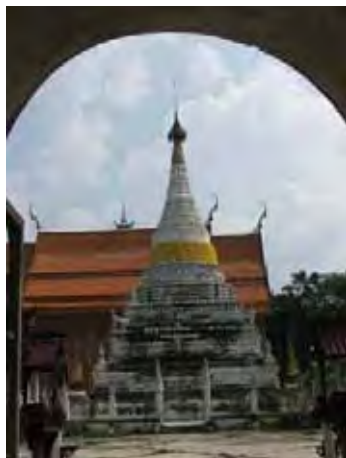
Figure 201: General condition of pagoda.
