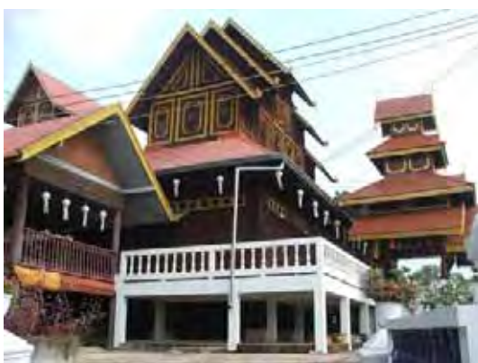
Figure 211: Condition of the monastery. (Photograph: 07.11.2008)
