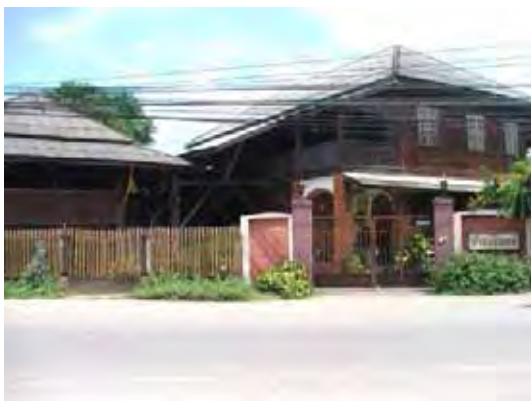
Figure 156: Bombay House. ( Photograph: 07.07.2009 )
