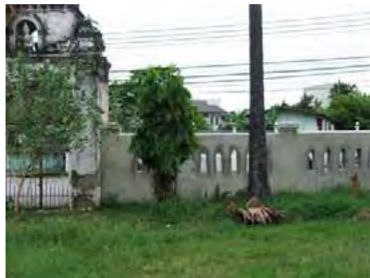
Figure 204: The reconstructed wall. (Photograph: 29.03.2009)
