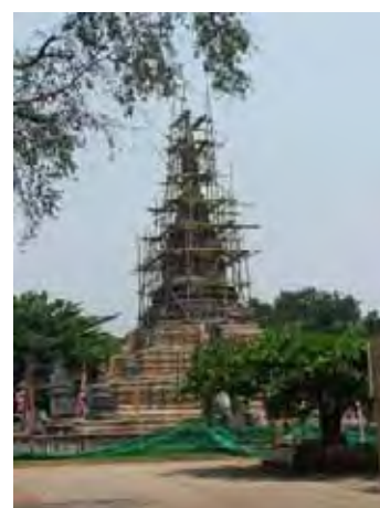
Figure 124: The pagoda in the process of renovation.
