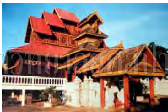
Figure 207: Condition of the monastery before restoration by Fine Arts Department.
