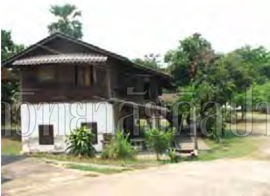
Figure 112: The typical half wood and masonry building as a monk's living cell. ( Photograph: 29.03.2009 )
