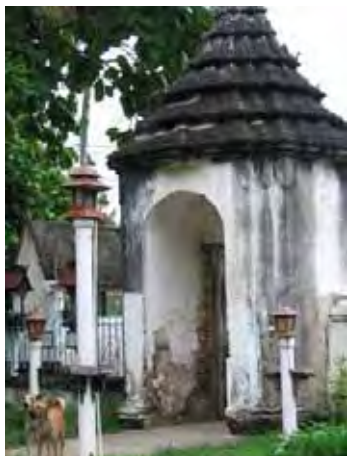
Figure 203: Condition of gatehouse. (Photograph: 29.03.2009)
