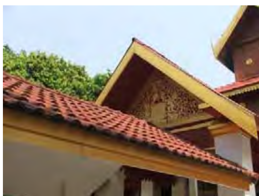
Figure 180: Condition of a gable of a new main hall (vihara).
