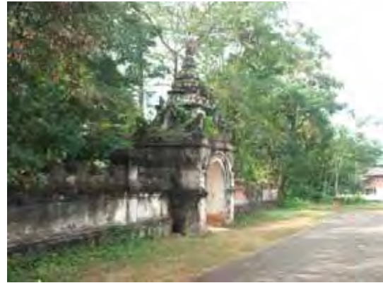
Figure 106: The porch entrance gate.
