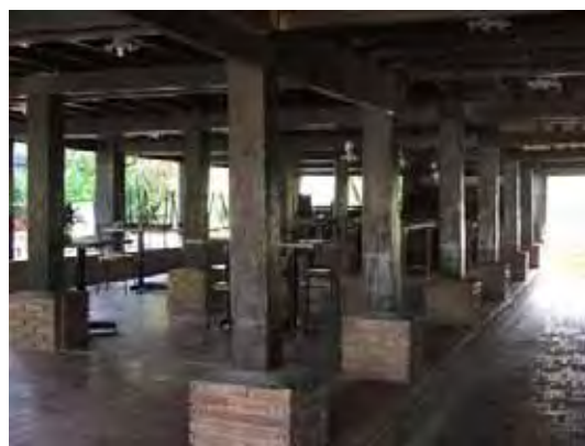
Figure 235: Addition of concrete plinths.
