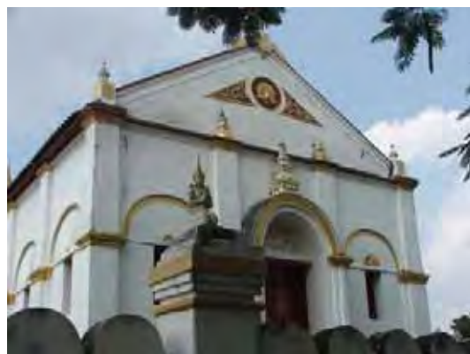
Figure 214: Condition of the vihara.
