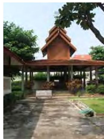
Figure 70: View of Zayat. ( Photograph: 17.11.2008 )
