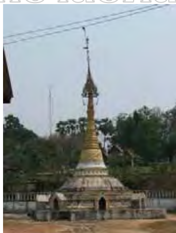
Figure 229: Condition of pagoda. ( Photograph: 29.03.2009 )
