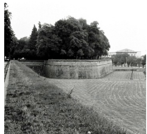
View of the orillon of a bastion at Lucca, seen from the rampart
