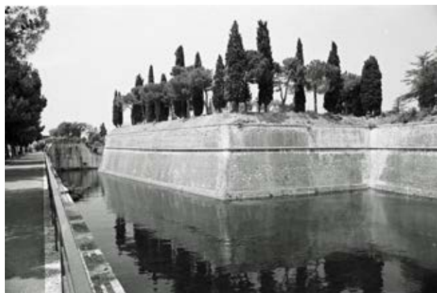
View of a bastion without orillon at Peschiera del Garda
