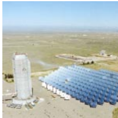
The National Solar Thermal Test Facility in Albuquerque, New Mexico, USA
