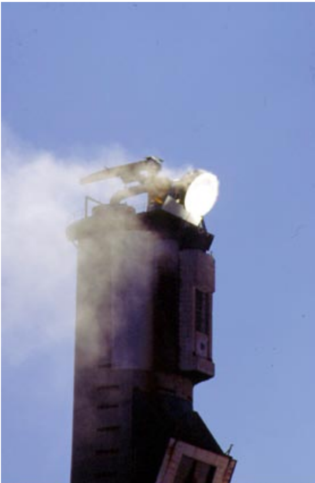
TSA Power Tower Testing at Plataforma Solar de Almería
