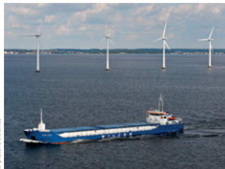
An off-shore wind farm in the Sound off Copenhagen, Denmark
