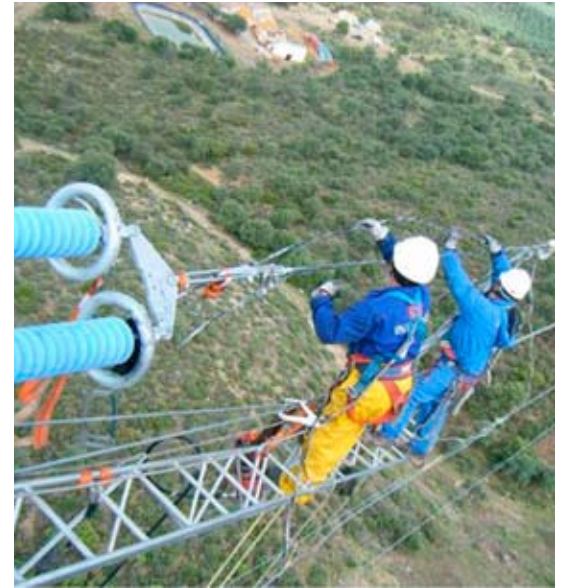
HTLS Installation Process
