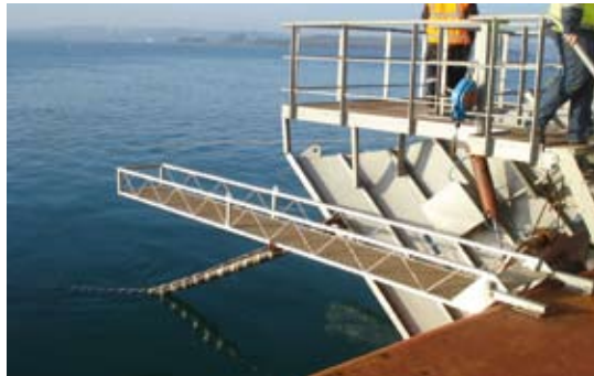
Submarine cable laying in shipping lane
