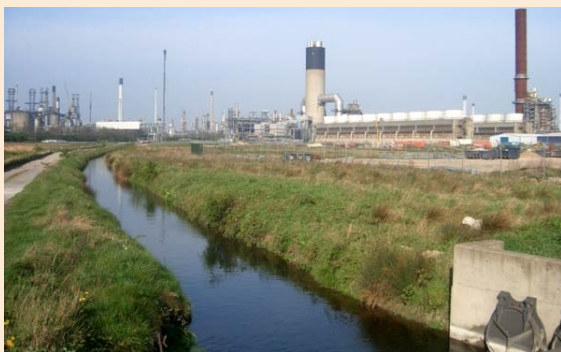
South Killingholme Drain and Immingham Power Plant
