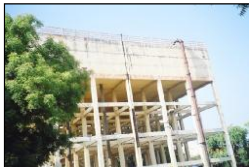
Overhead Tank at Cruzpuram
