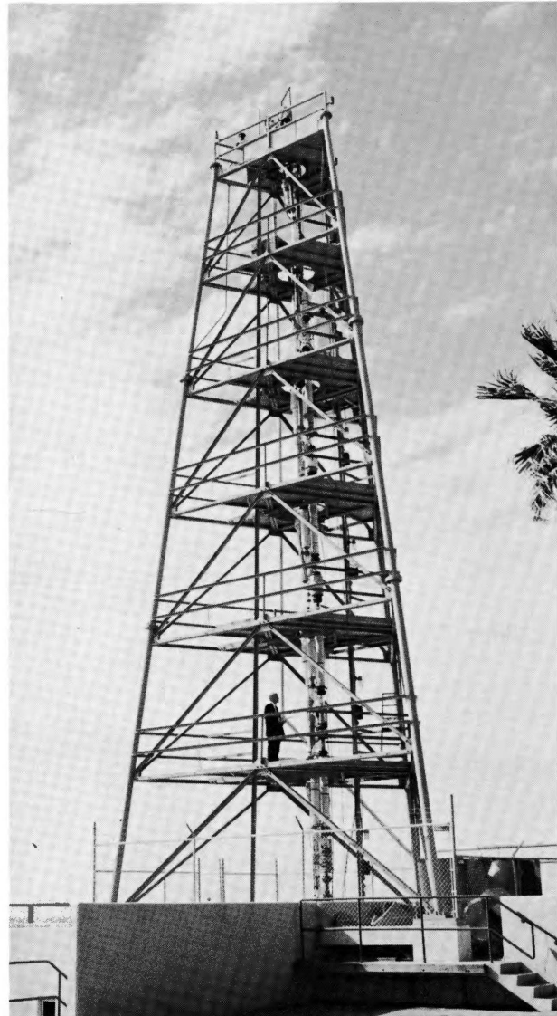
Multiple-effect flash evaporator system utilizes 90-foot tower in desalination study financed by State of California.
