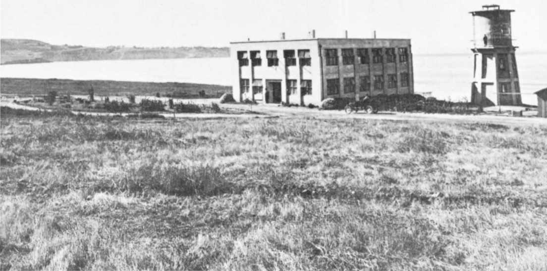
George H. Scripps building just completed in 1910, still in use in 1966.
