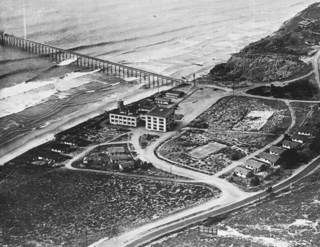
The Scripps Building, (center left, above) became the nucleus of a complex of buildings which by 1916 included the museum library (joined to the Scripps Building by a bridge), the aquarium (behind the two larger buildings above), the pier, the Director's home (on the triangle of land, above right) and housing for visitors and staff scattered over the hillside.
