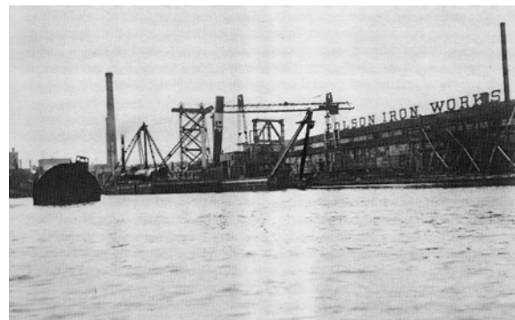
Figure 22: Knapp's Roller Boat rusting in the Frederick Street Slip, September 1914 (from Stinson and Moir 1991:5).
