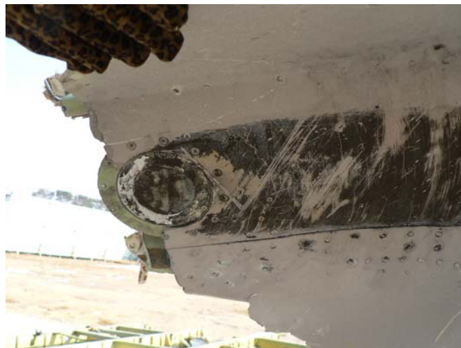
[Figure 19] Exterior Skin of the Cockpit Smoke Evacuation Shutter
