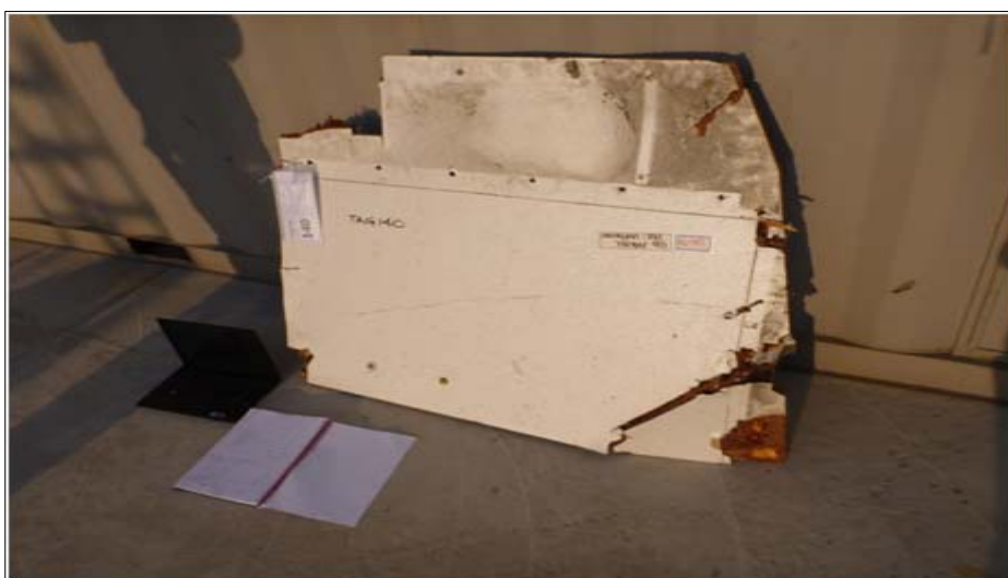
[Figure 37] Upper Deck Interior Panel with Area of Sooting
