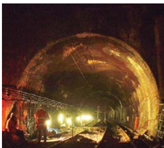
Smart Infrastructure team conducting work in tunnel, February 2006
