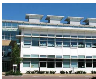
Building using the E-Stack system for natural ventilation: Aldwyck Housing, Luton, UK
