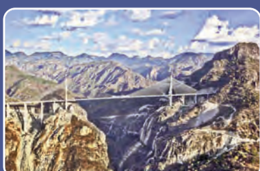
The world's highest suspension bridge
