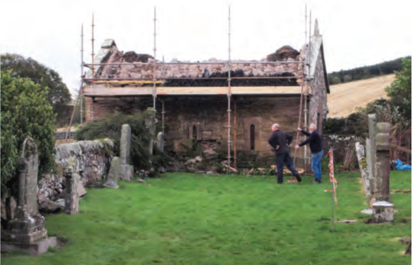
The stone barrel-vault was stabilised and the roof replaced.
