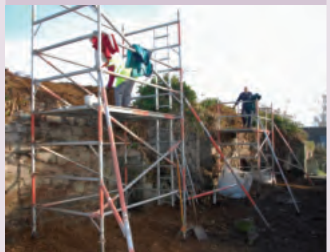
Clearing the wall-heads in February 2012.
