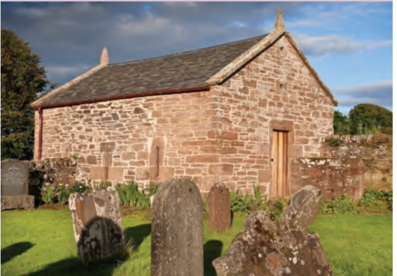
Conservation work substantially completed by late March 2012 (© George Logan)
