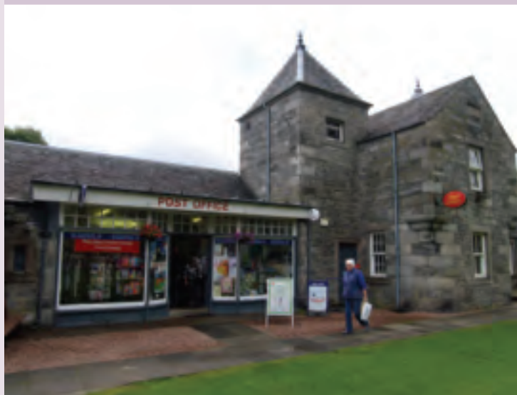
The Conservation Area Regeneration Scheme (supported by Historic Scotland) will see fabric repairs to several properties in Blair Atholl.
