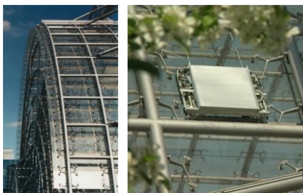
Figure 2. The Leipzig Fair building and the robot at work on the glass surface.
