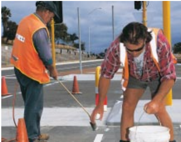
Adding final touches to Reid Highway.
