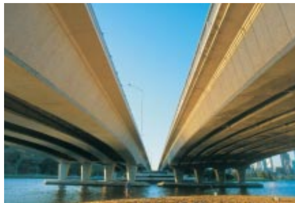
The duplicated Narrows Bridge.
