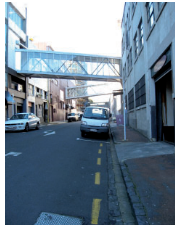
Figure XXIII Cross Street overbridges
