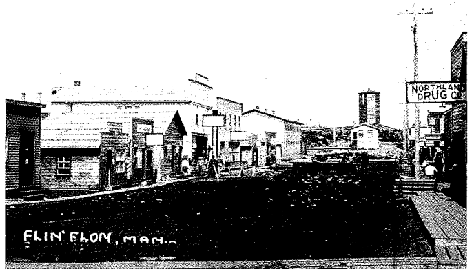
By the fall of 1931 drainage ditches had been installed along Main Street alleviating the water problem. (S. Strandland)
