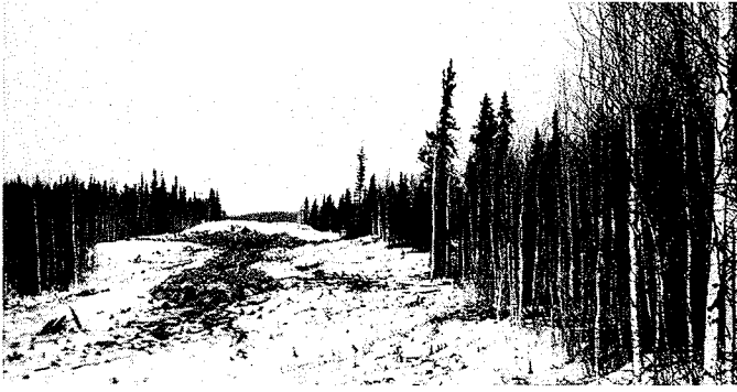
The many lakes along the RAILWAY ROUTE from Cranberry Portage to Flin Flon allowed access to several different points for clearing and grading ahead of the steel. (H. Guymer 1928)
