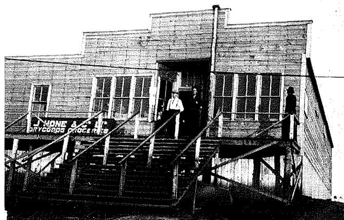
Jack Hone replaced his first log store with this modern 74' x 66' building situated just west of the company staffhouse. (F. A. Hollier 1929)
