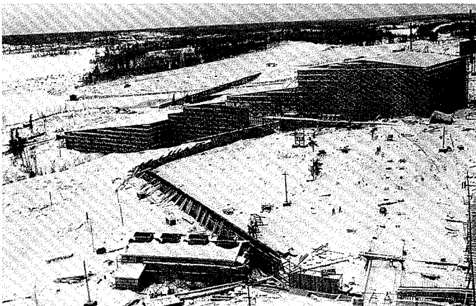
The mill steel almost completed. (H. Ennis 1929)
