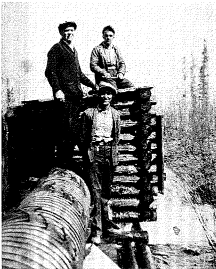
Working on the pipe line from Cliff Lake to the reservoir. Ole Wick, left, Vic Bowes and Les Foster. (Babe McCullum 1929)
