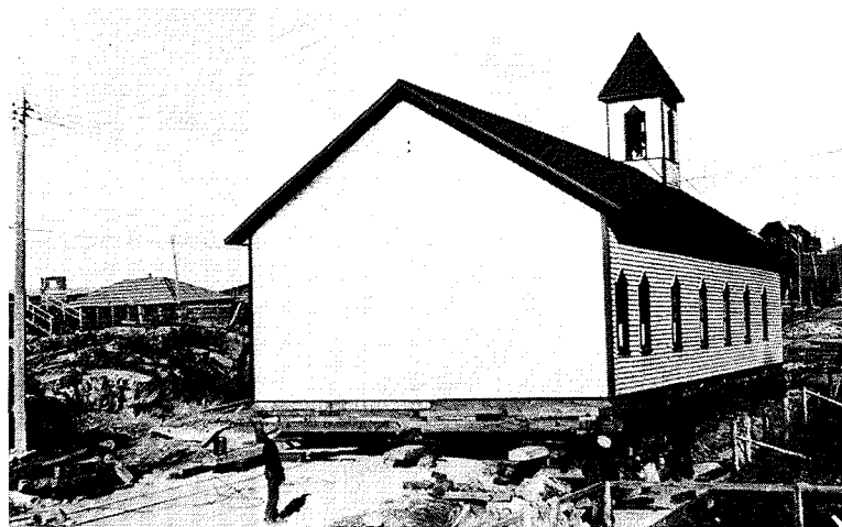
St. Augustine's Church being moved across Church Street to the lot formerly occupied by G. B. Mainwaring's residence. Mainwaring's house was moved to the former church site beside the Salvation Army Hall. St. Augustine was dedicated to St. Ann in October 1935. (J. Paylor September 1934)
