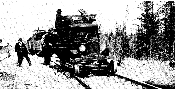
The Dominion Construction Company converted this car for easier transportation from one construction site to another. (F. A. Hollier 1928)
