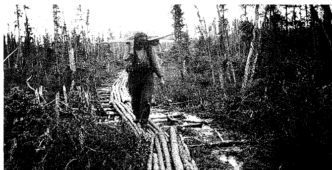
When nothing else was available, foot transportation on poles over the many stretches of muskeg was necessary between Wabishkok and Kiskeynew Lakes on the way to Island Falls. (H. Ennis 1928)
