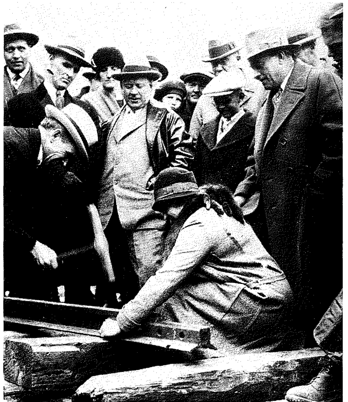
Mrs. Harry McLean holds the Golden Spike for Premier John Bracken at the completion of the line to Flin Flon in October 1928. Harry McLean, construction superintendent and Barney M. Stitt, M.P. for the Nelson Constituency look on. (H. Guymer)
