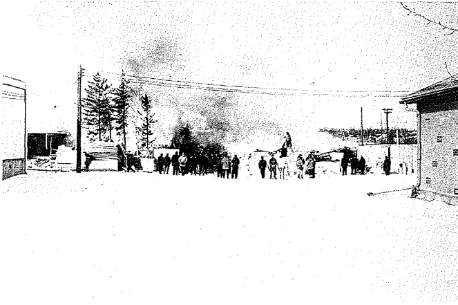
Fire at the Manor housing project, 1971. (Reminder)
