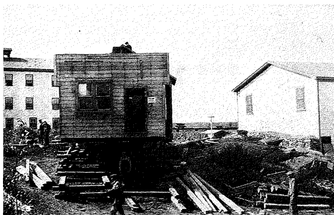
Construction of Hudson Bay Mining and Smelting required that the Northland Drug store be moved over to the townsite. (F. A. Hollier 1929)
