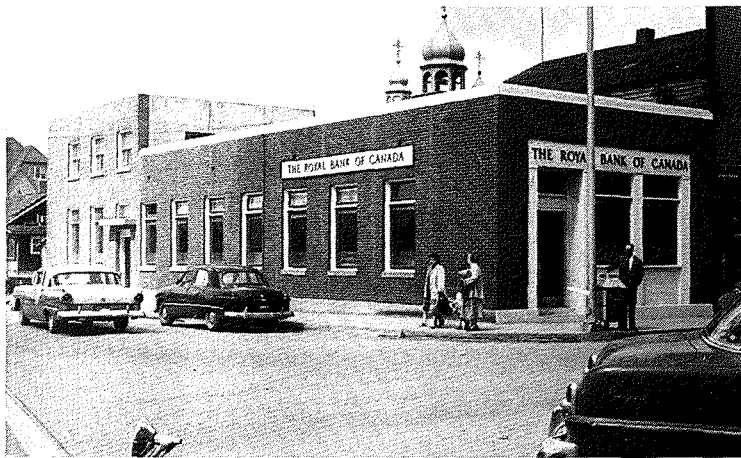
Royal Bank Building. (Royal Bank)
