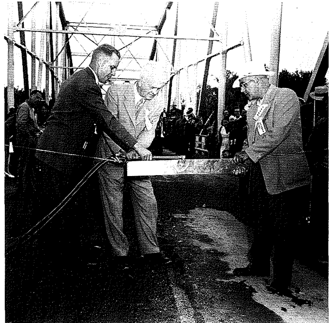
Lieut. Gov. the Hon. R. F. McWilliams cuts copper ribbon held by F. Wildgoose of Can. Liquid Air and Mayor C. Steventon, to officially open No. 10 Highway, Bakers' Narrows, July 11, 1951. (Reminder)
