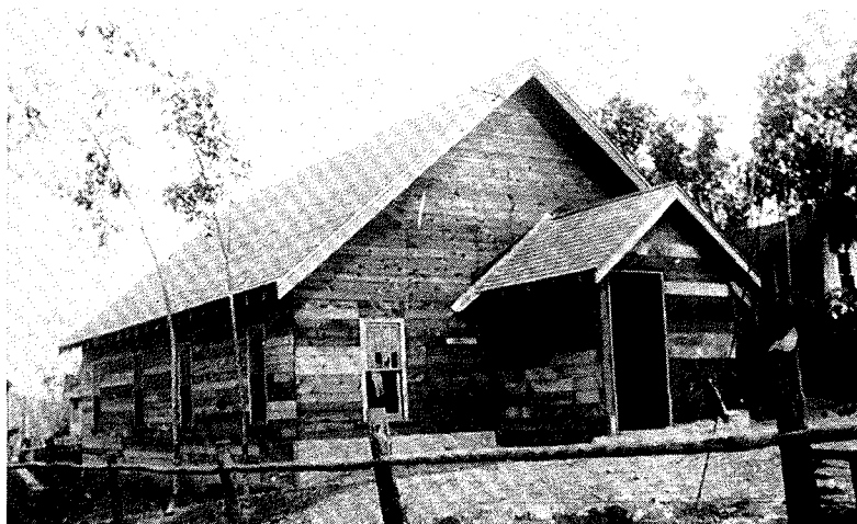
First Pentecostal Church was built in 1935. (Pentecostal Church)
