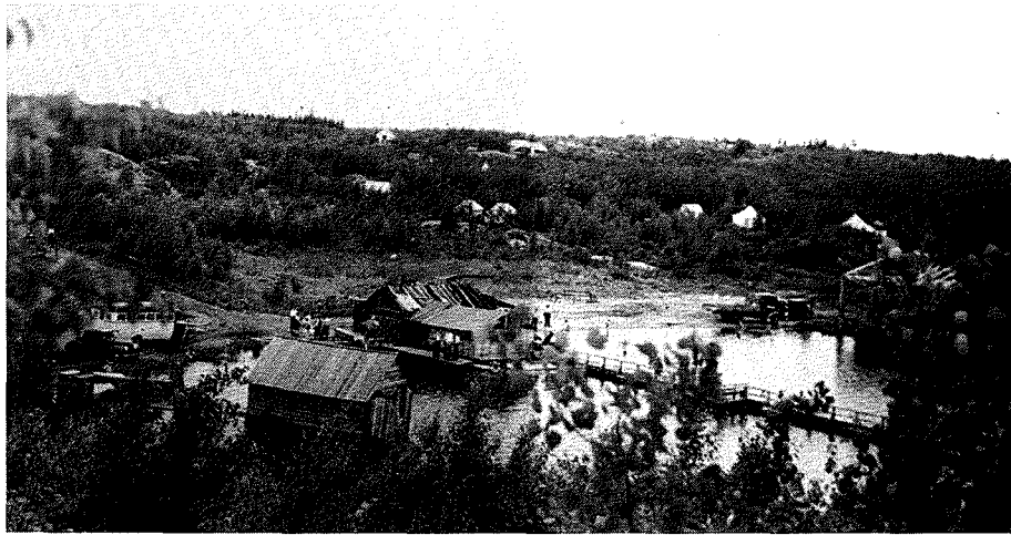
Phantom Lake in 1932 provided summer recreation for the people of Flin Flon. Paddy Faubert's dance hall under construction far right. (K. Allen)
