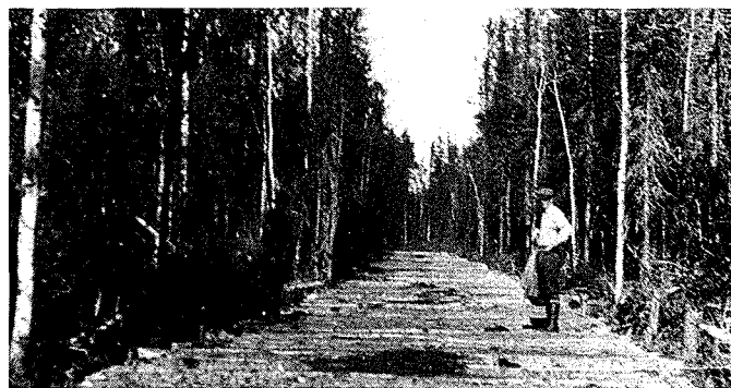
Logs were laid side by side over muskeg areas to create a 'corduroy' road. (Manitoba Archives 1925)
