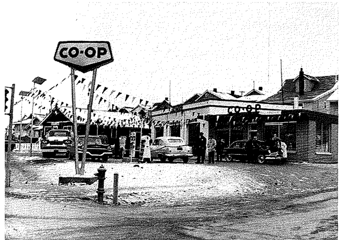
The COOP Garage came later. (Reminder)
