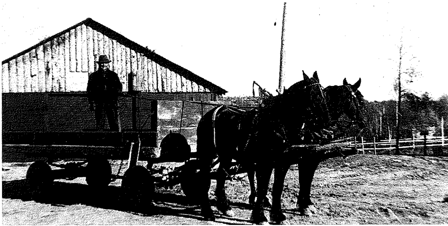
Harold Leask started his draying service in Flin Flon in 1934. He moved from the Halfway on the Phantom Lake Road to the Barn Area in 1937. (B. Leask)
