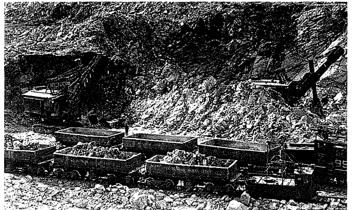
Electric Marian shovels loaded the loose rock into the 22 yard side dump cars for delivery to the crusher. (Flin Flon Historical Society 1931)
