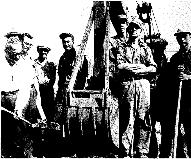
Town Public Works and Utilities prepare for sewer and water in east Birchview with Mayor Freedman turning first shovel of dirt. Looking on are Andy Watson, Dick Evans, Charlie Hagen, Ernie Ransom, Bob Comstock and Henry Hartle, July 26, 1955. (Reminder)
