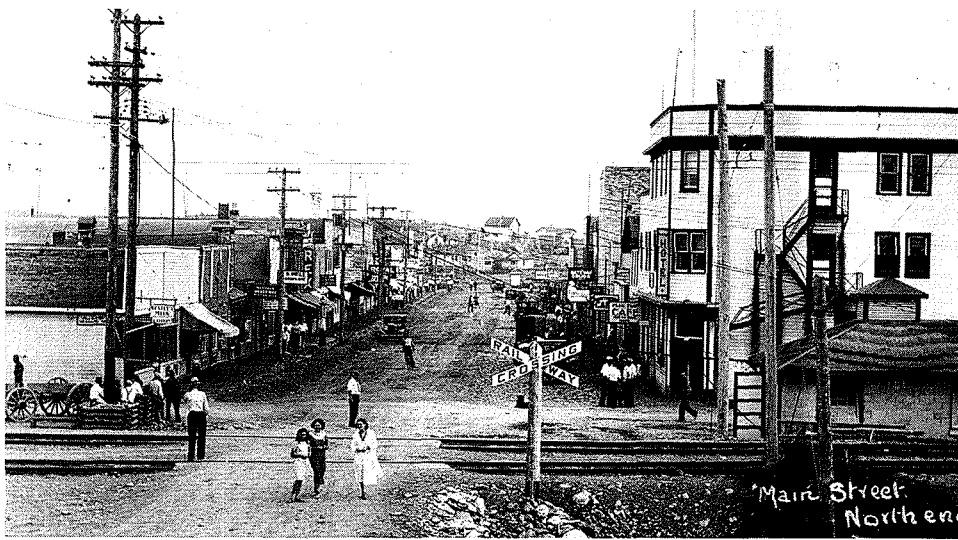
North end of Main Street — sidewalks were completed and the roadway built up with gravel. (Babe McCullum 1936)
