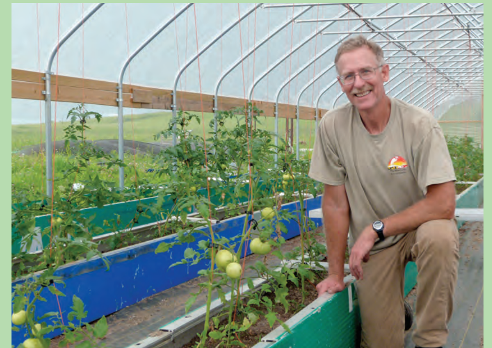
Construction of the Frostburg Grows greenhouse is well underway. Paul used old highway signs to make the raised beds, water storage tanks and parts of the greenhouse itself.
