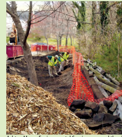
Ashton Manor Environmental Services prepped the site.
