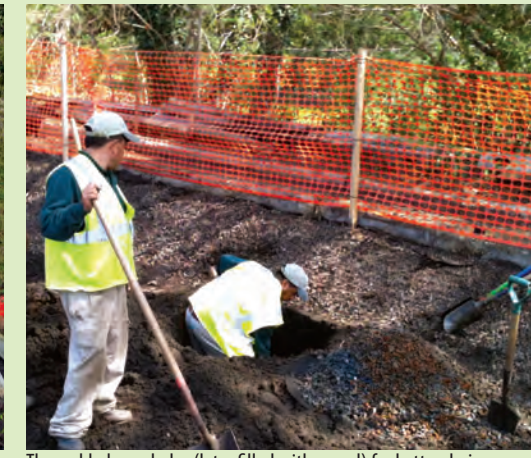
They added new holes (later filled with gravel) for better drainage.
