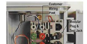
The device itself will have 3-5 posts that interconnect the telecommunications company's wire to your inside wire. If the NID is located outside your house, it will have a plastic cover. You will need to remove this cover to access the wiring, but since this cover is an important protector of the telephone equipment, it must be properly reinstalled after your work is completed. The telephone company side of the NID is locked and you should not attempt to open it.
