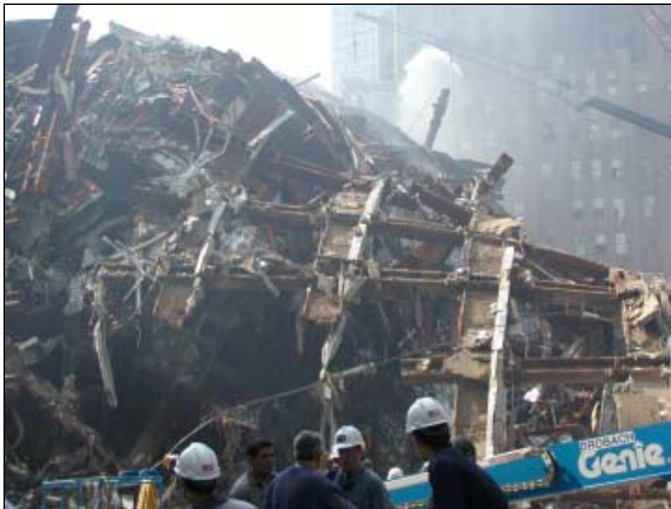
Figure 3.13. Portions of conventional steel moment-resisting frames were observed in the debris pile
