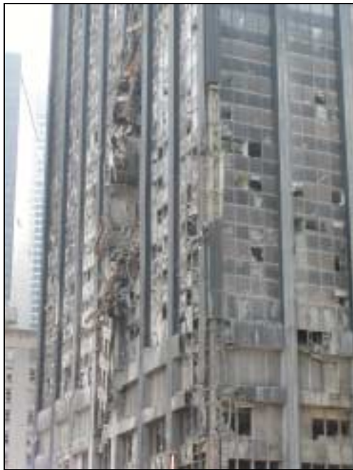
Figure 3.25. Twenty story gash in the north façade of the building, from the 26 th to the 6 th story
