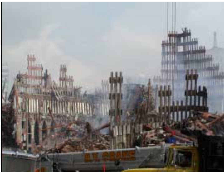
Figure 3.5. (continued). Portions of the perimeter tubes of WTC 1 and 2 that remained standing in the debris pile (as of September 21, 2001)
