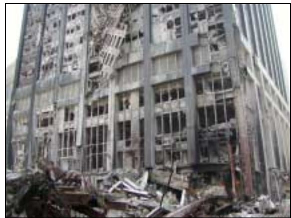
Figure 3.25. Twenty story gash in the north façade of the building, from the 26 th to the 6 th story
