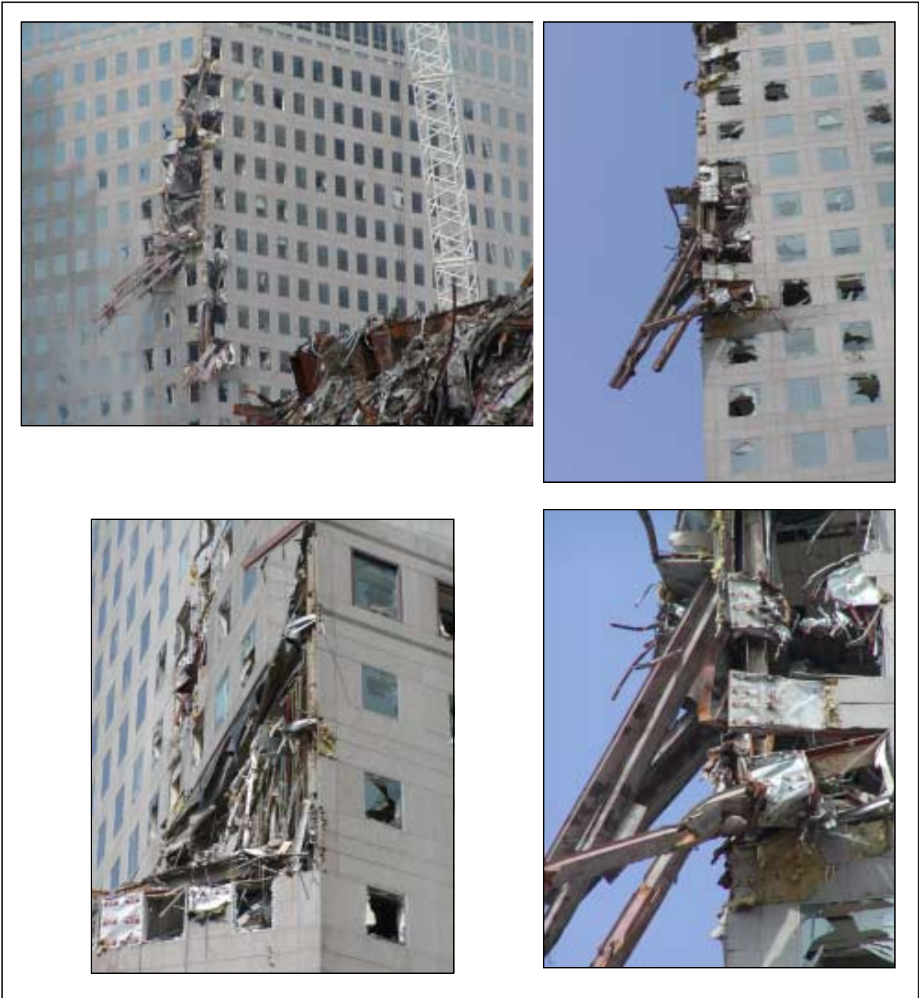
Figure 3.20. (continued) Damage to the façade of 3 World Financial Center
