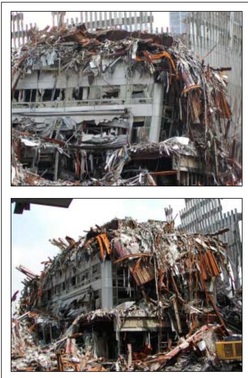
Figure 3.8. Debris falling destroyed WTC 3
