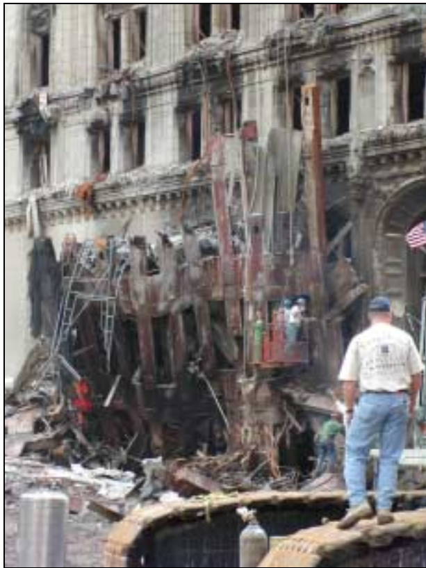
Figure 3.23. Large multi-ton segment of the façade of the WTC 2 lodged at base of the 90 West Street building
