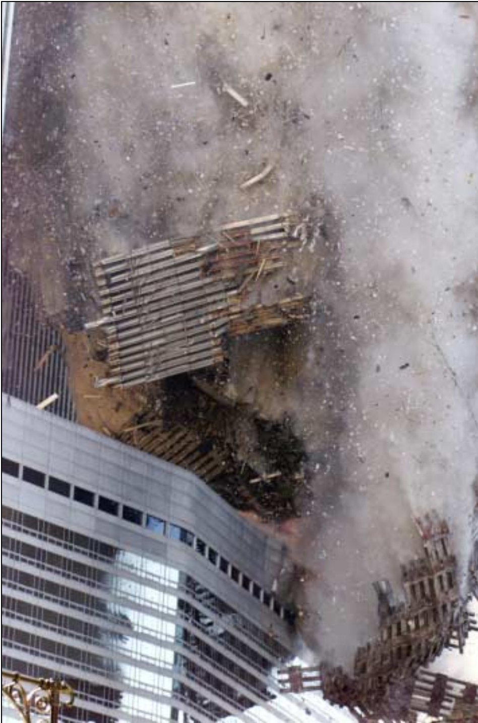
Figure 2.2. Large segments of the World Trade Center perimeter frame fell on adjacent buildings during the collapse of the towers
