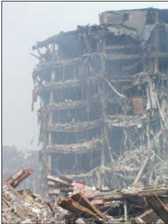
Figure 3.9. (continued). Falling and burning debris destroyed WTC 4
