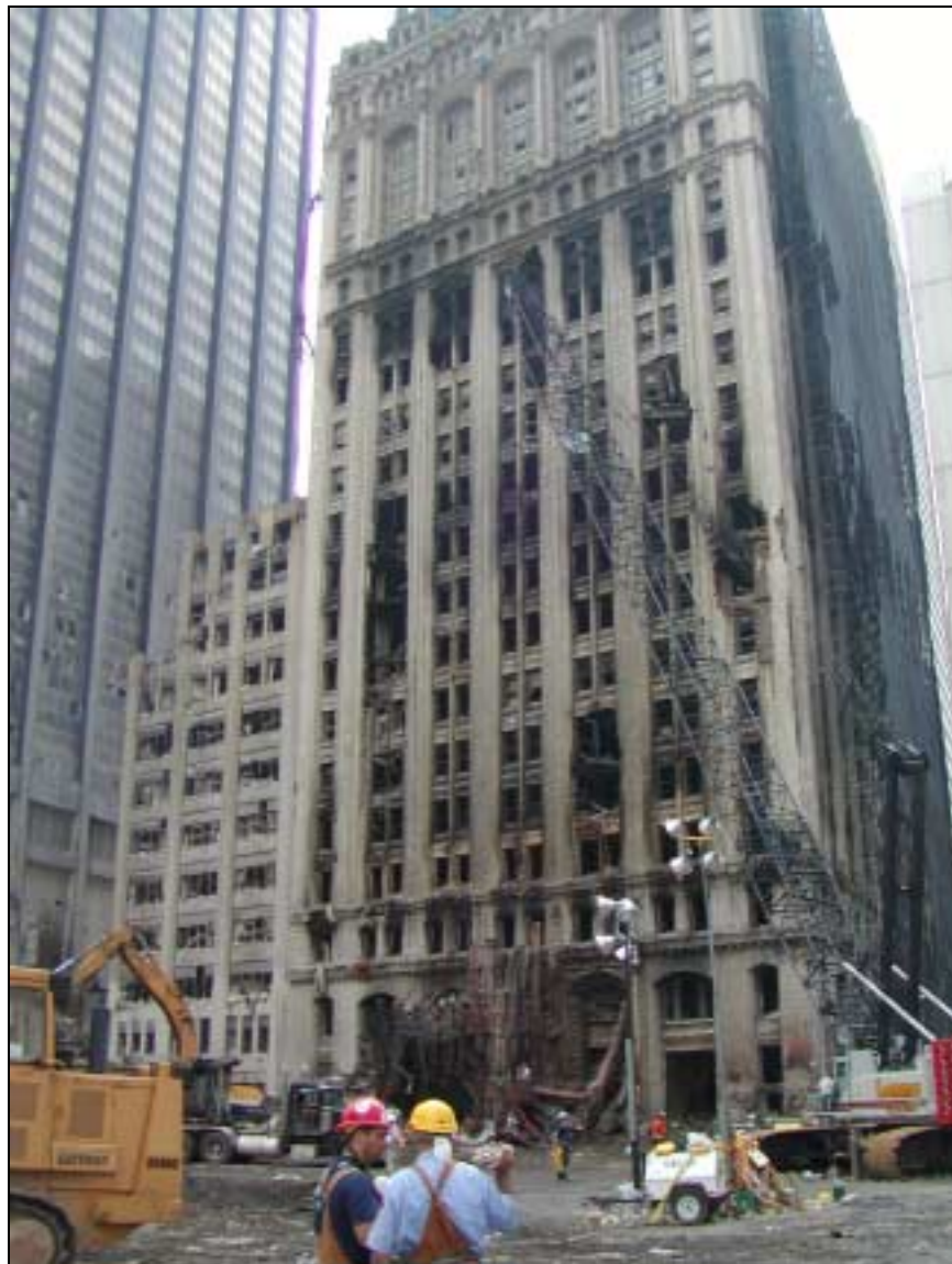
Figure 3.22. 90 West Street building
