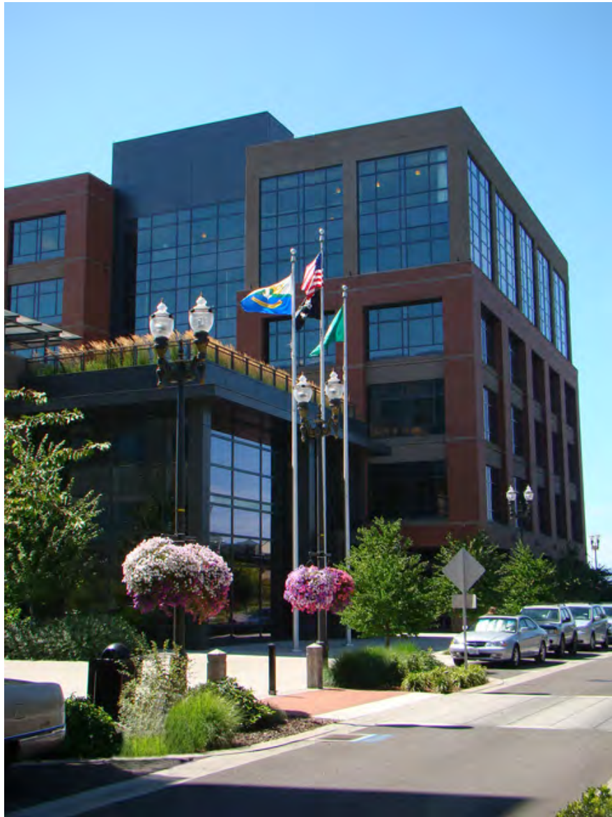
City Hall, 415 W 6 th Street
