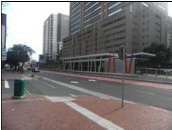
Photograph 7.3: IRT Thibault Bus Stations , ARG Architects
