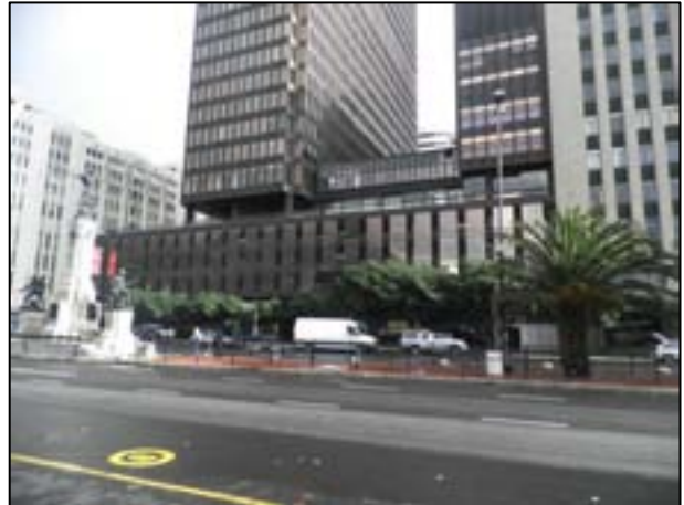
Photograph 3.31: Adderley street between Riebeeck and Strand streets , O'Donoghue 2012
