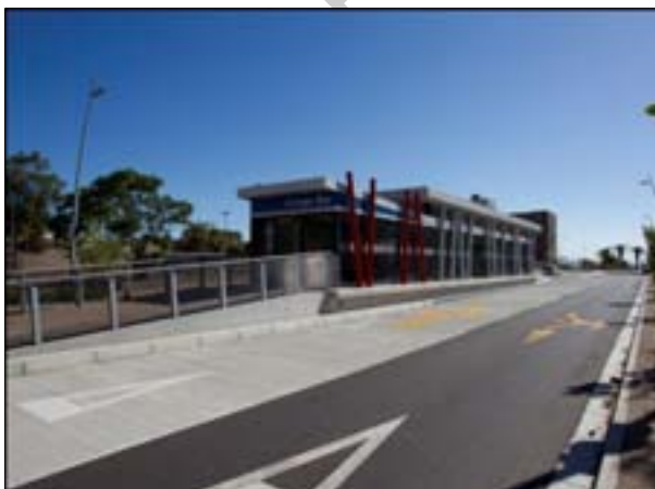
Photograph 7.5: IRT Green Point Bus Station , entry point from access ramp, ARG Architects
