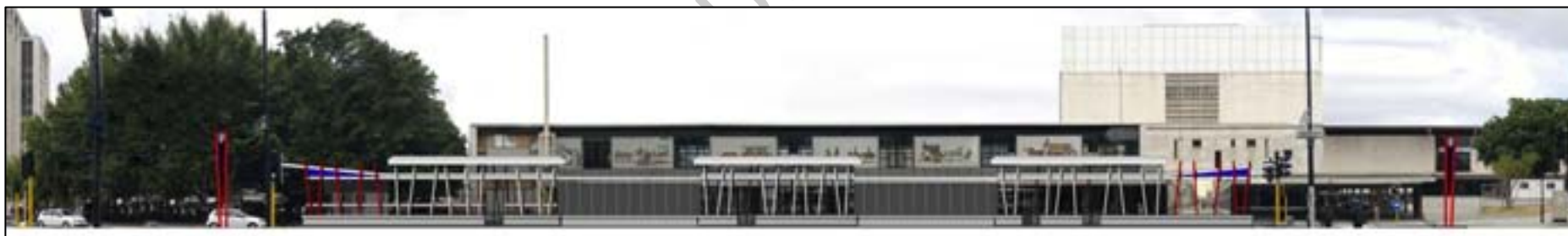
Image 7.2: Adderley IRT Bus Station East Elevation with the Railway Station in the background, ARG Design 2012
