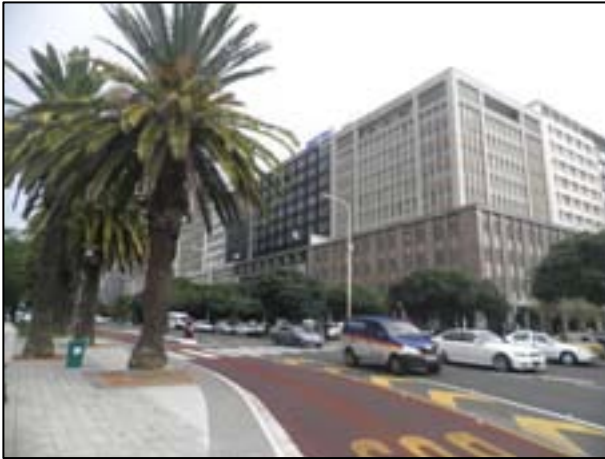
Photograph 3.46: Buildings bordering upper Heerengracht on north west boundary, O'Donoghue 2011
