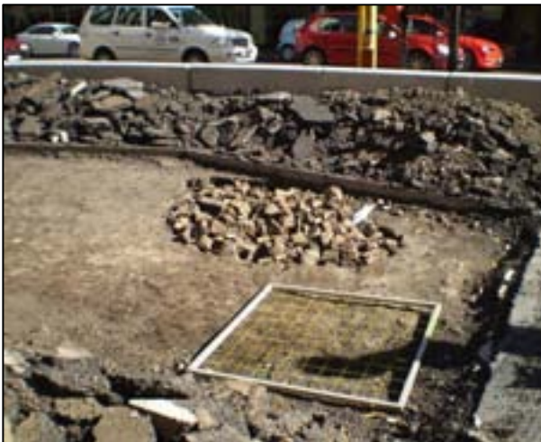
Photograph 3.20: Adderley street former surface: Wooden sets discover in 2010 during the construction of the cycle lane, O'Donoghue 2010
