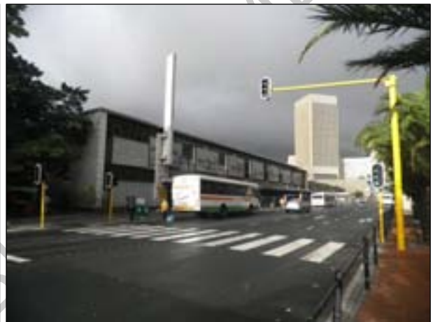
Photograph 3.39: Cape Town railway station complex, completed in 1961, and covered between 25 and 35 city blocks. It underwent a major renovation in 2009/2010;
