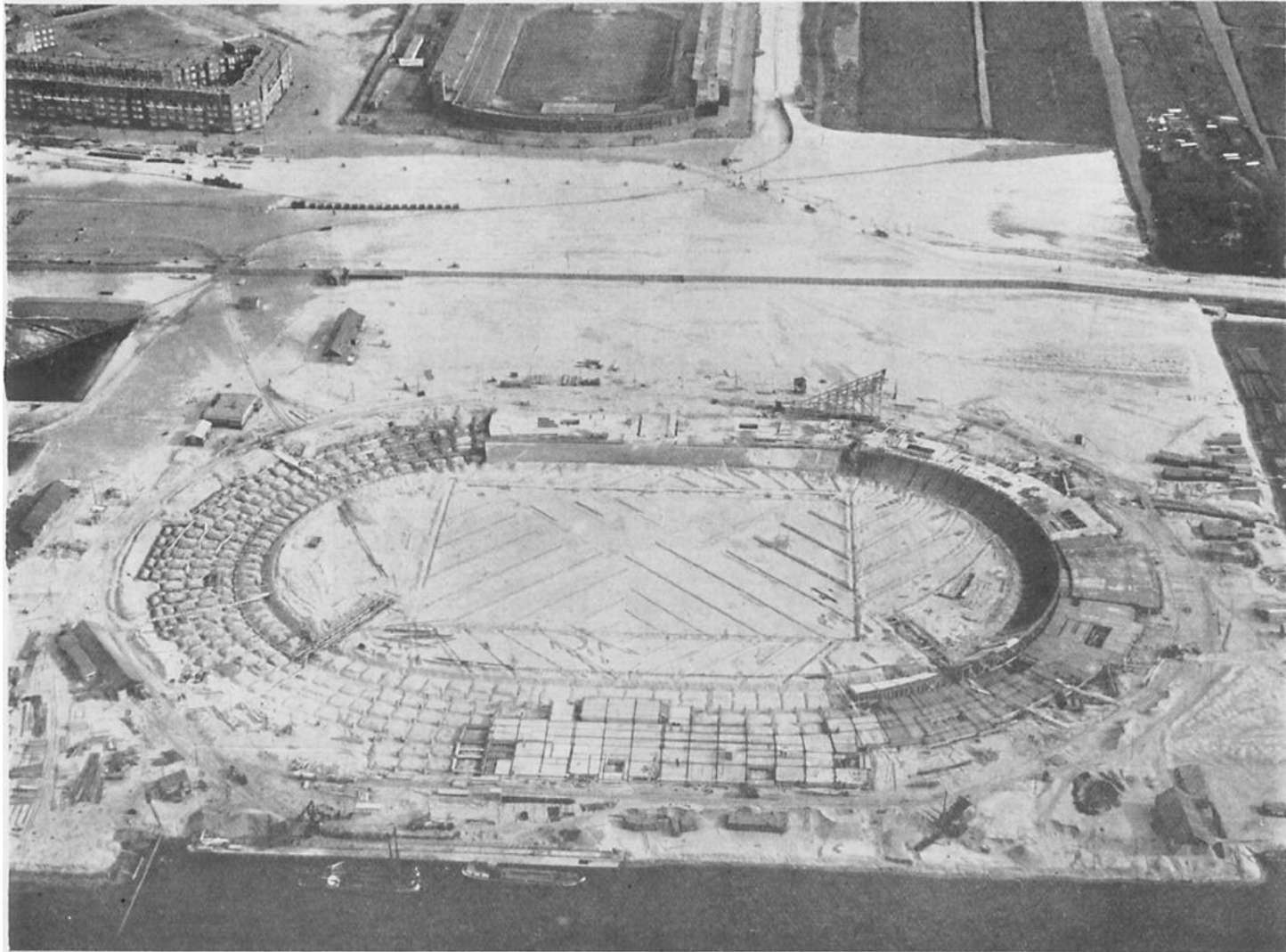
Bird's-eye view of the Stadium in the course of construction.
