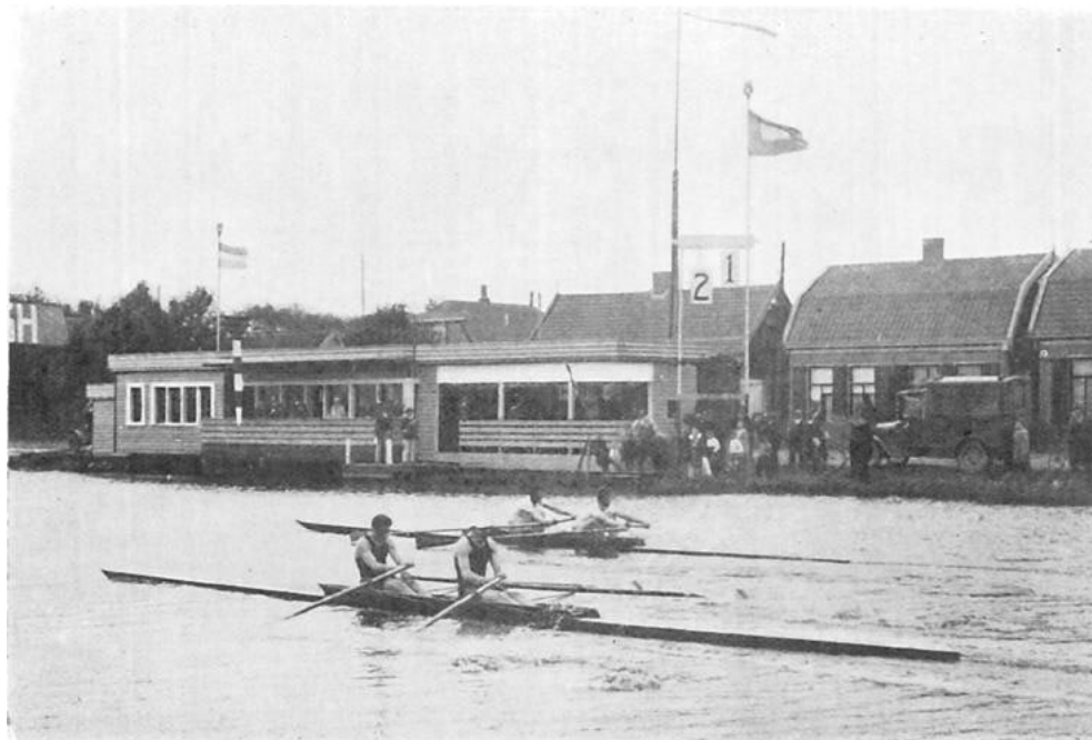
Double Scull. The building in the background accommodated the jury.
