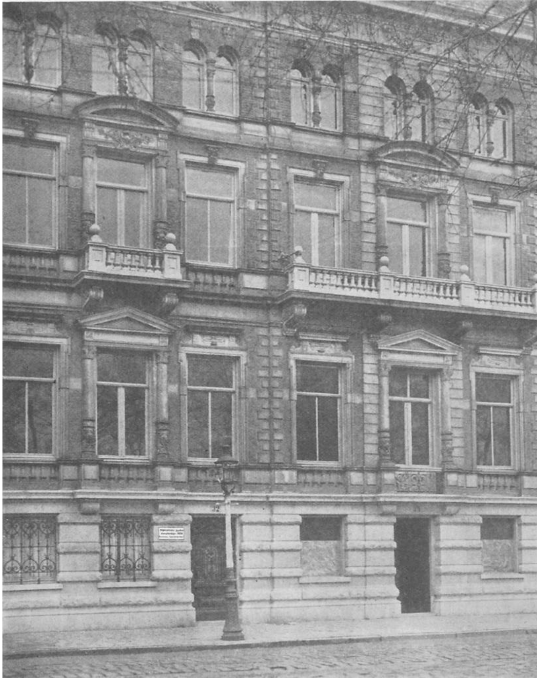
The houses Weesperzijde 32 and 33 at Amsterdam, where the offices were located.
