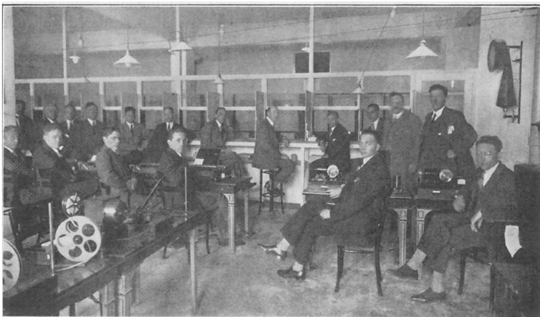
The transmitting room behind the counter.
