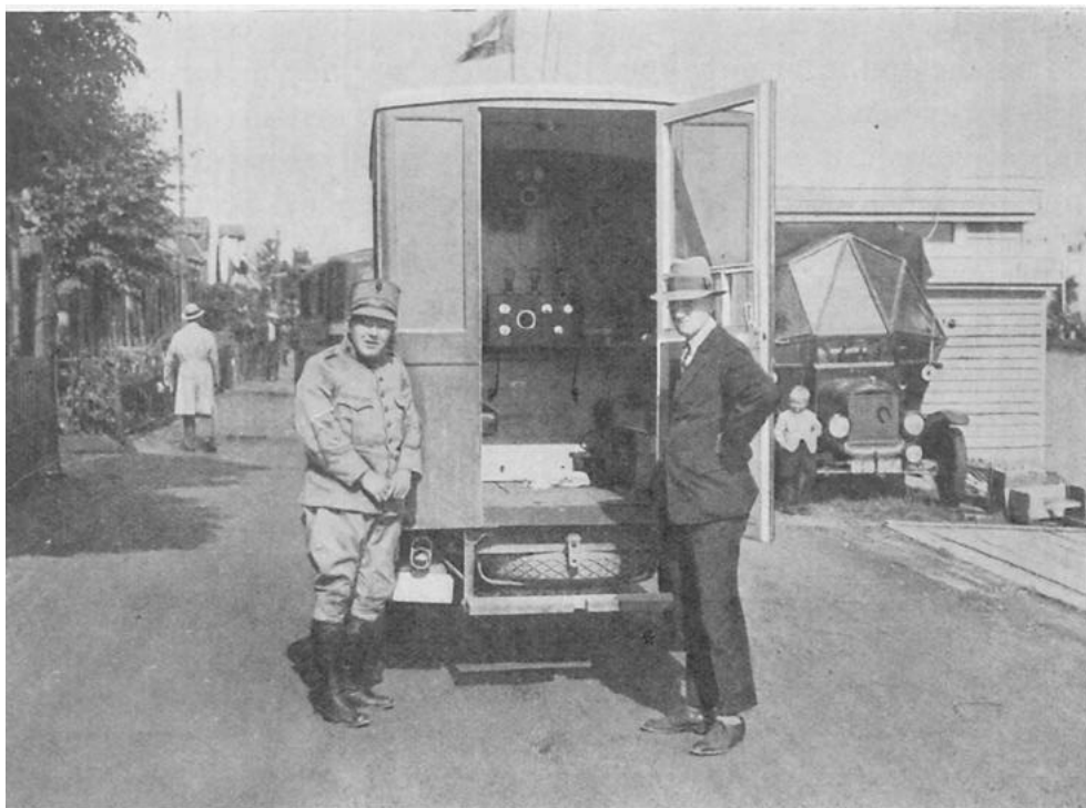
The loud-speaker installation at Sloten.
