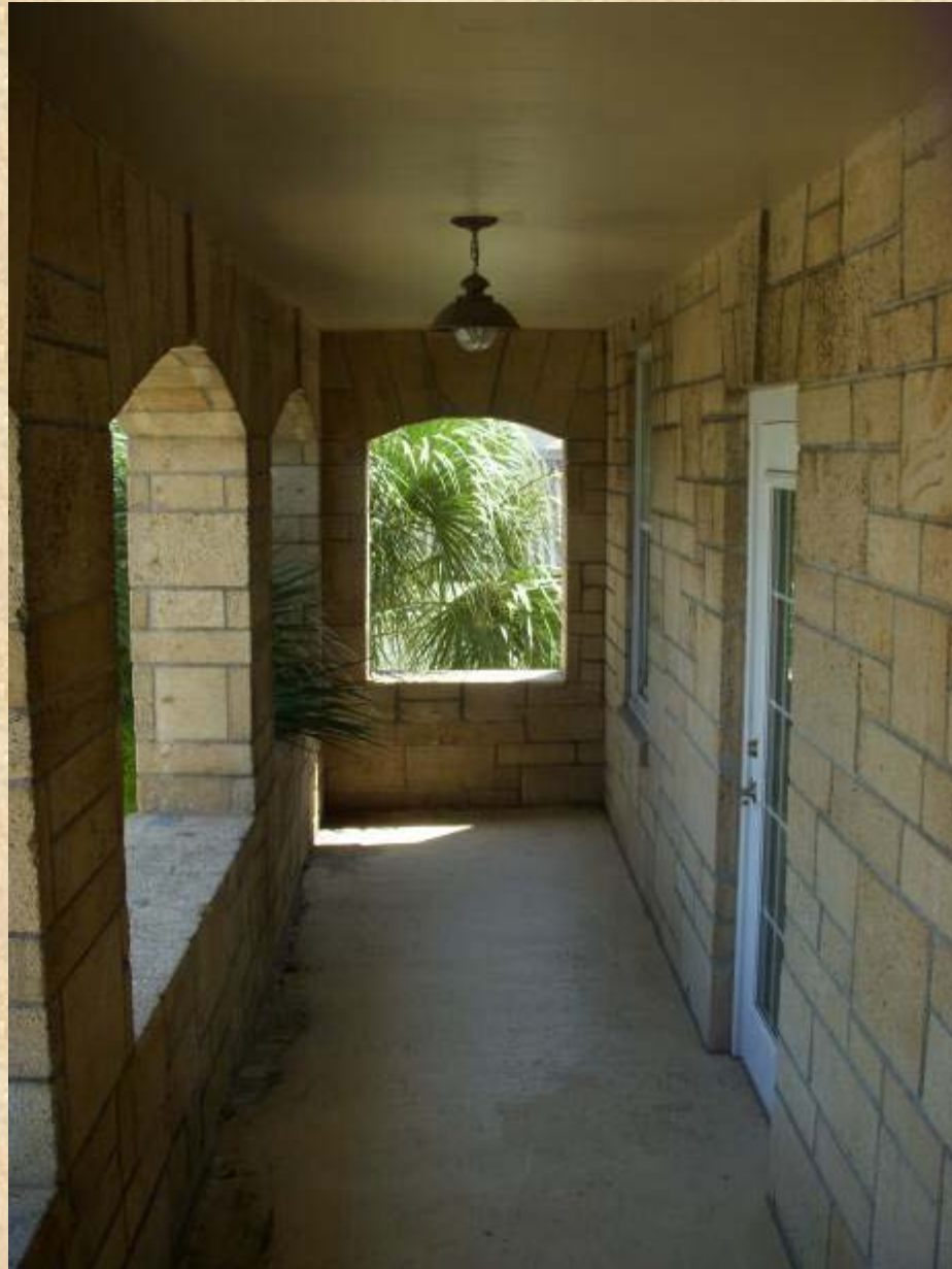
Ormond Beach Fire House
