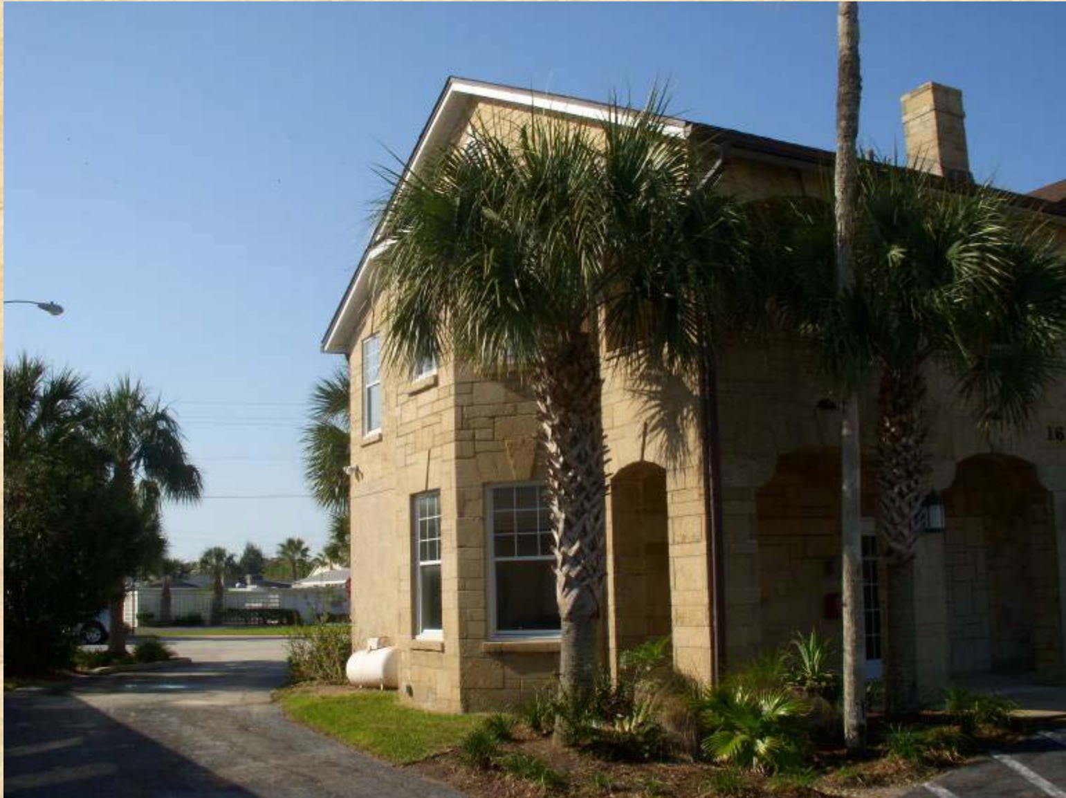
Ormond Beach Fire House
