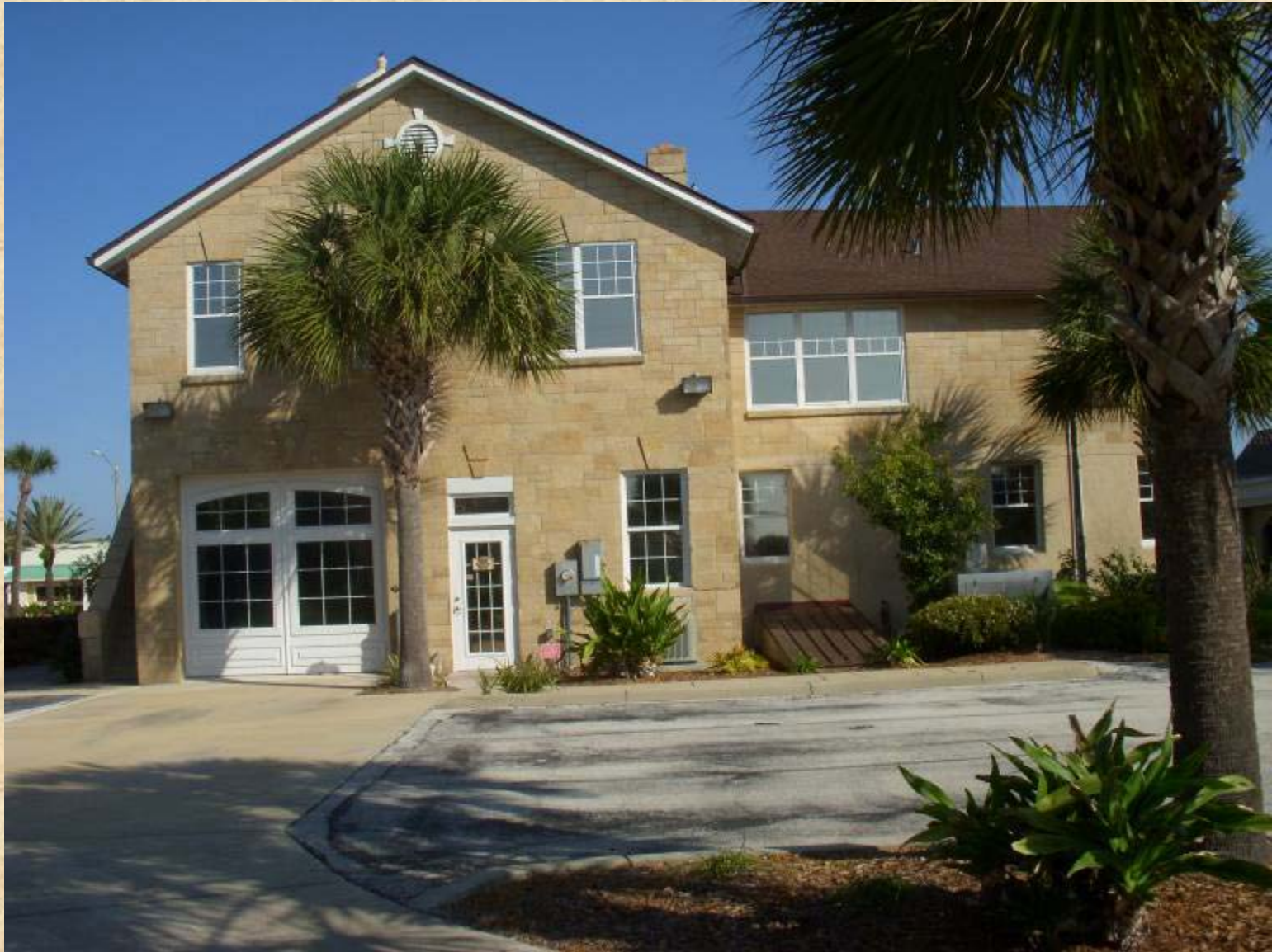
Ormond Beach Fire House
