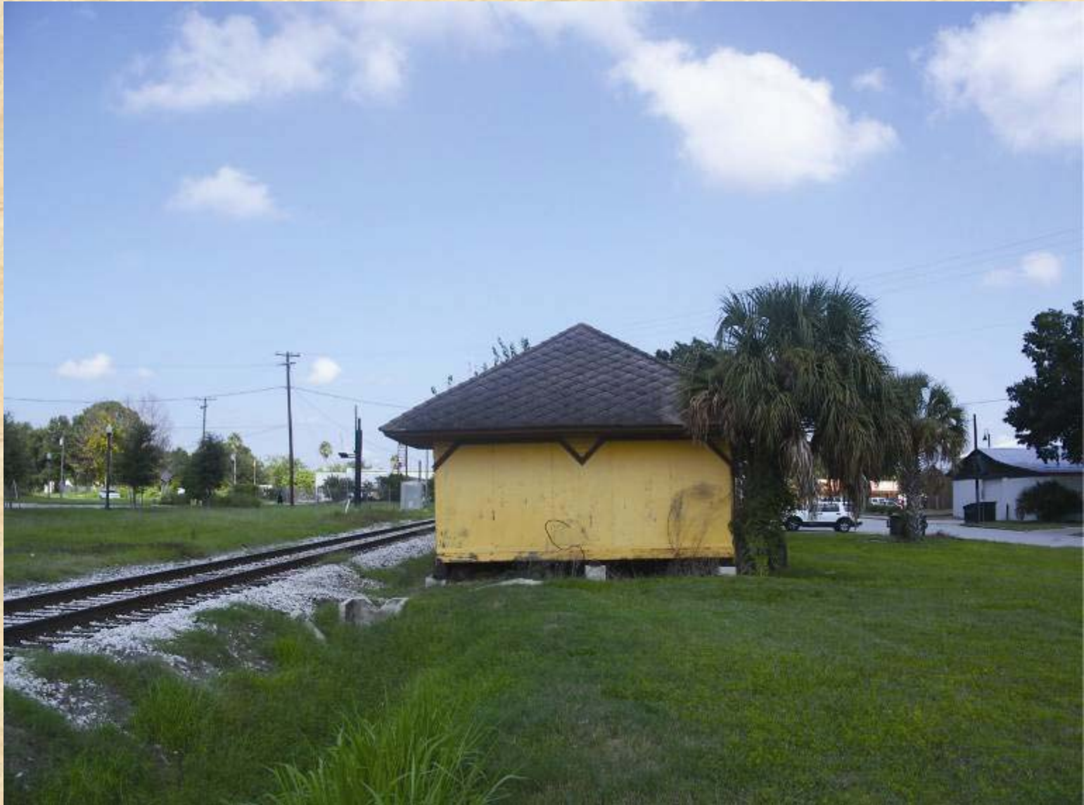
Apopka Seaboard Air Line Railroad Depot
