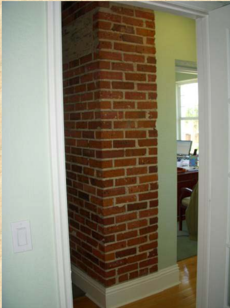
Ormond Beach Fire House
