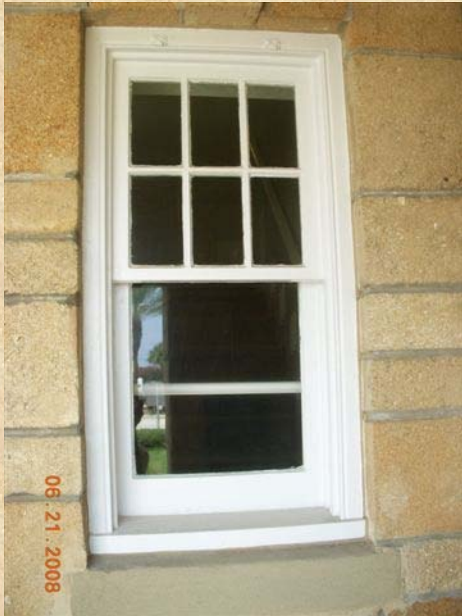
Ormond Beach Fire House
