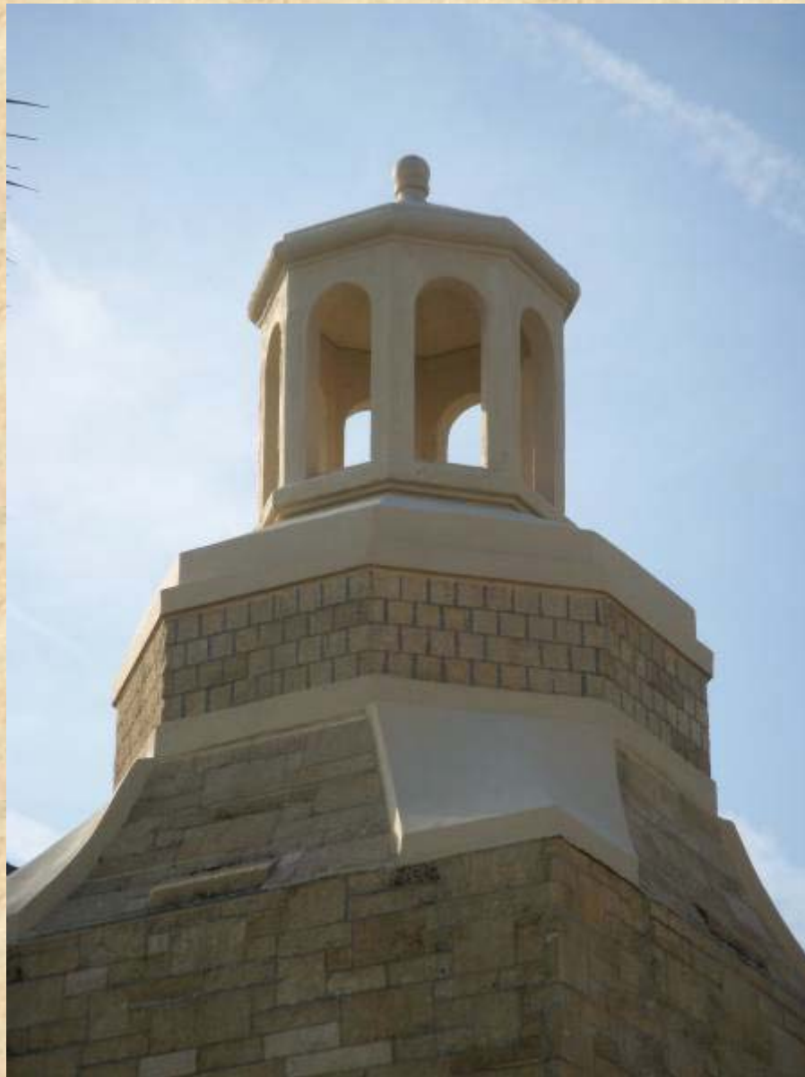
Ormond Beach Fire House
