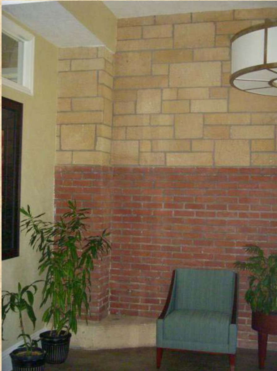
Ormond Beach Fire House
