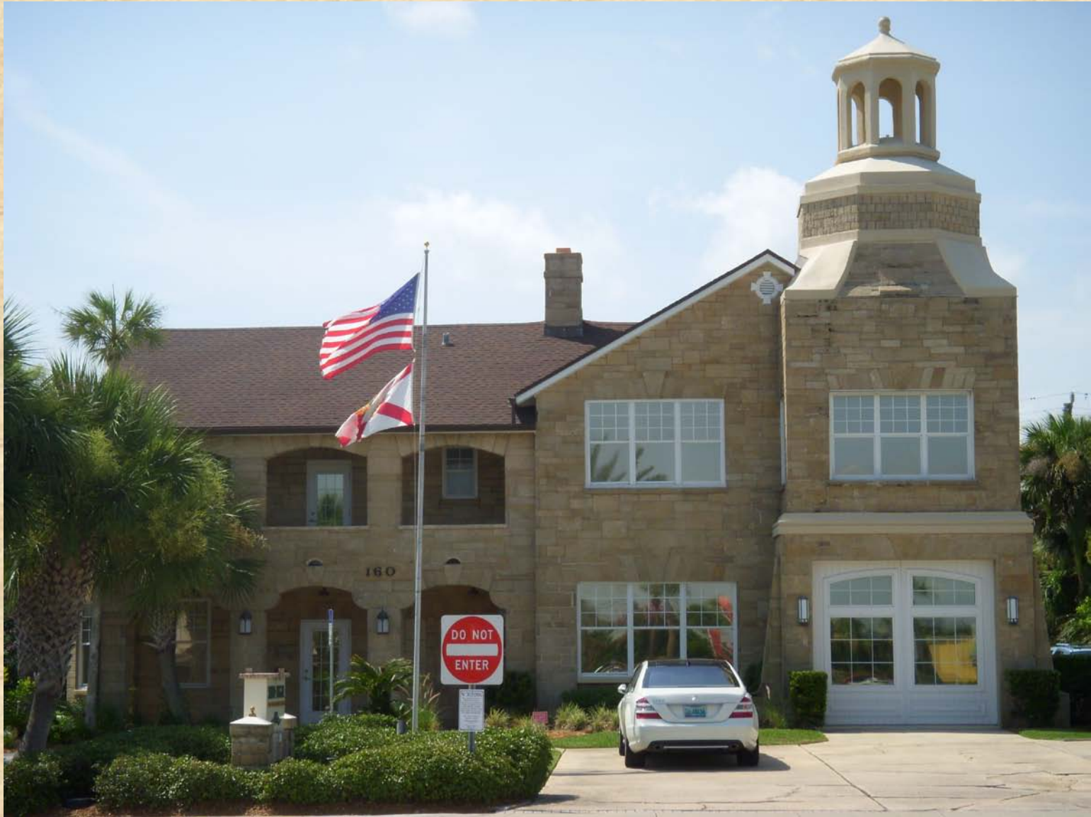
Ormond Beach Fire House
