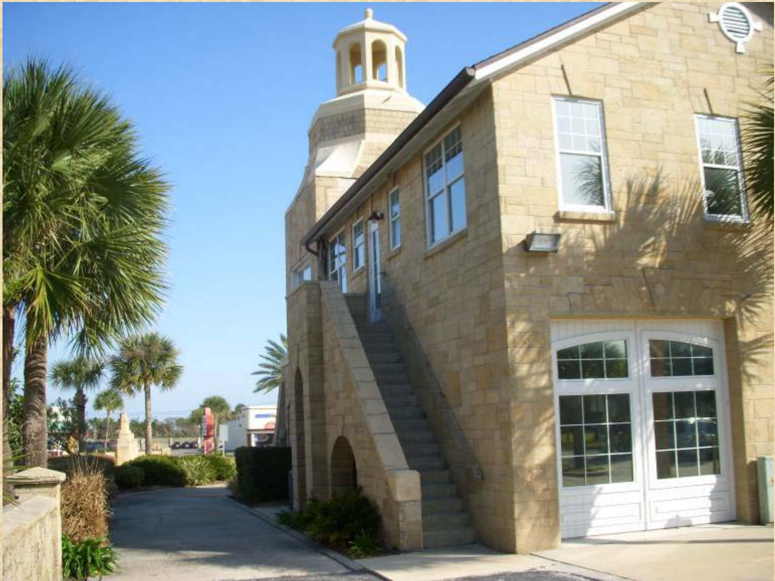
Ormond Beach Fire House
