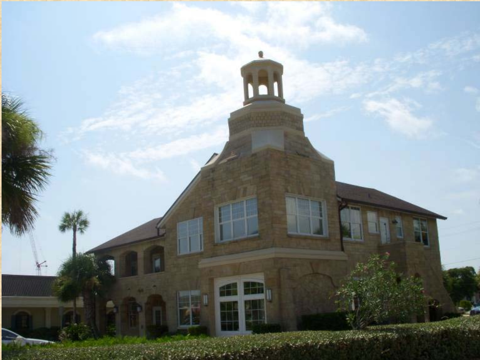
Ormond Beach Fire House
