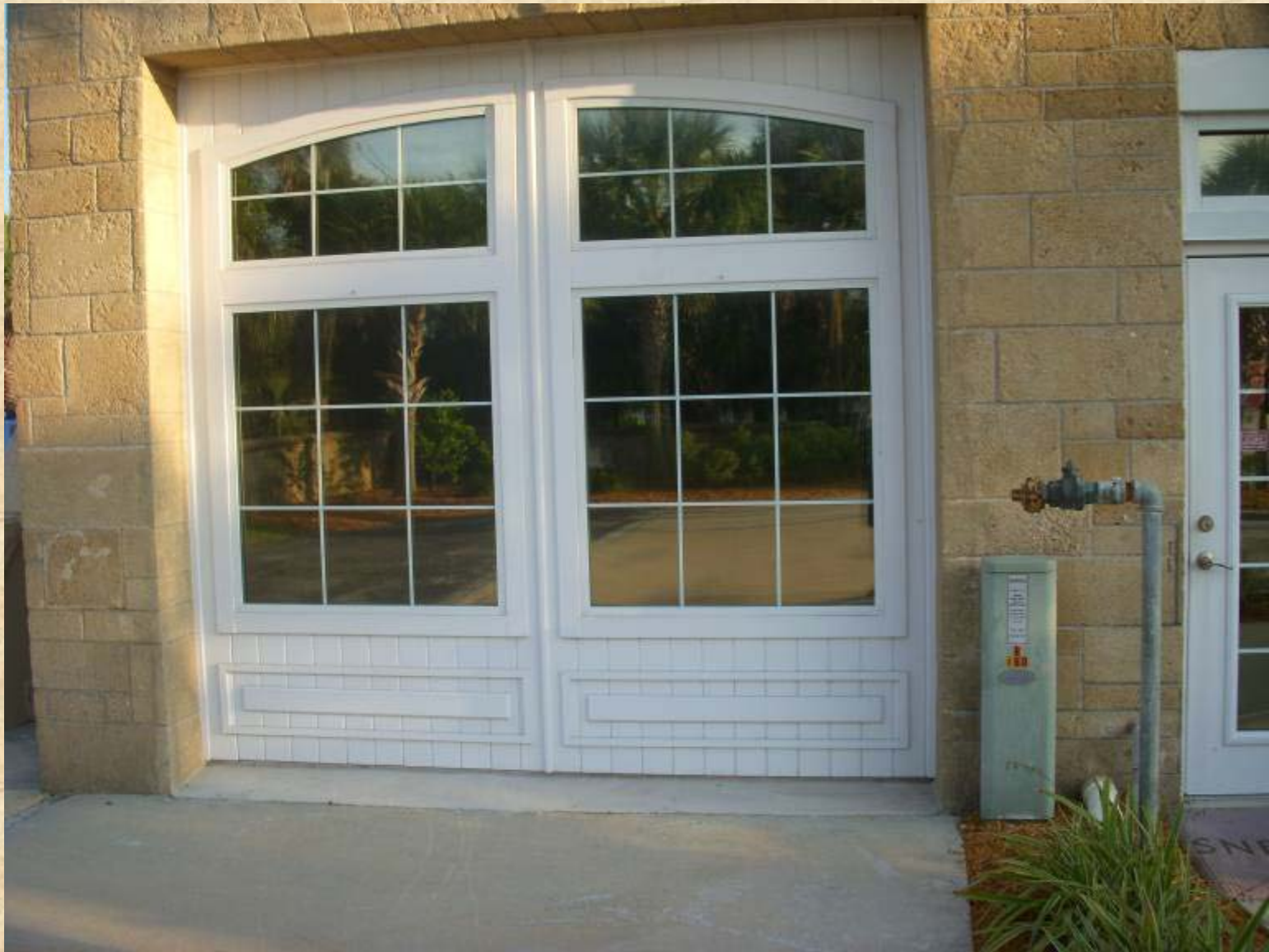
Ormond Beach Fire House
