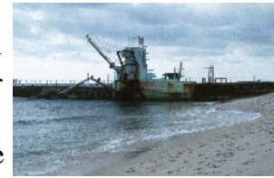
South Lake Worth Inlet Sand Transfer Plant
