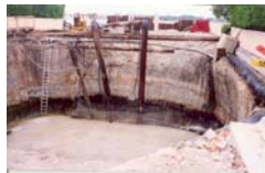
Town of Palm Beach Stormwater/D12 Wet Well Total Grant Award = $200,000
