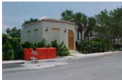
Town of Palm Beach Stormwater/D12 Pump Station Total Grant Award = $200,000
