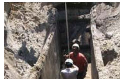
Hypoluxo Installation of Sewers (Septic Replacement) Total Grant Award = $450,000
