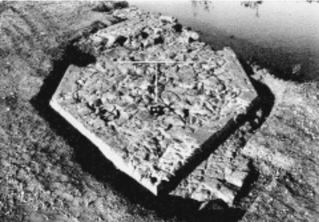
13th century bridge pier foundation, Hemington Quarry, Leicestershire (photograph: S. Ripper, University of Leicester Archaeological Services, © Leicestershire County Council)
