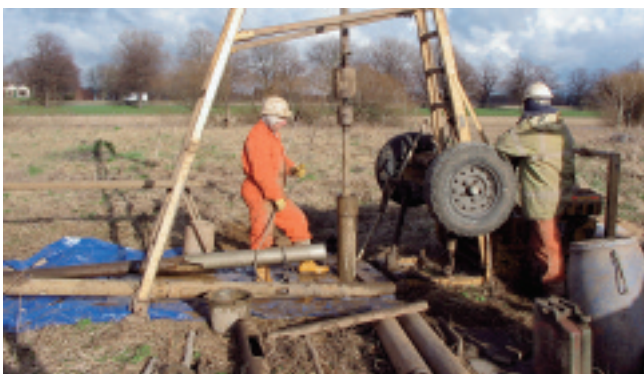
Borehole through alluvial deposits in the Trent floodplain near Clifton, Nottingham (photograph: P. Inker)
