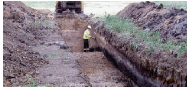
Late prehistoric palaeochannel at Hicken's Bridge, Aston-upon-Trent, Derbyshire; deposits of peat show as a dark wedge in the side of the excavation (photograph: A.J. Howard)
