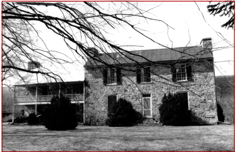
Oban Hall's 1825 architecture is well preserved to this day.
